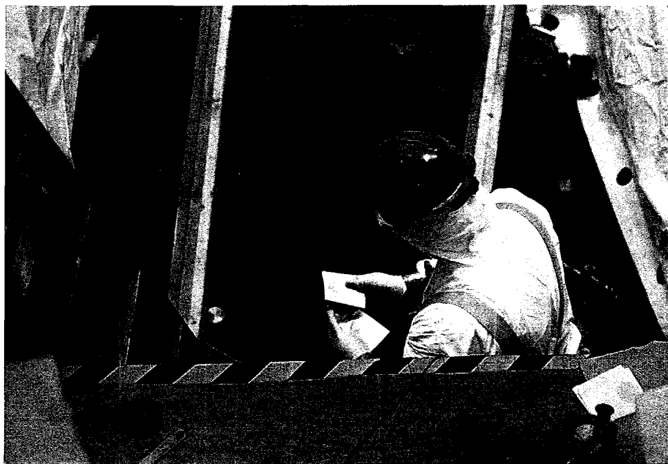
Figure 6.38 Health Physics Technician Surveying Graphite Prior to Removal (ANL Negative #23072K, Frame #9)
