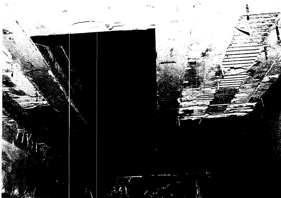
Figure 6.23 High-Dose Room Ceiling Partially Removed (ANL Negative #22981K, Frame #13)
