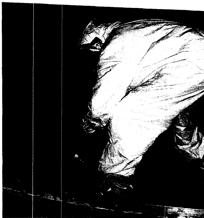
Figure 6.40 Technician Size Reducing a Section of Steel Shell for Packaging (ANL Negative #23407K, Frame #3A)
