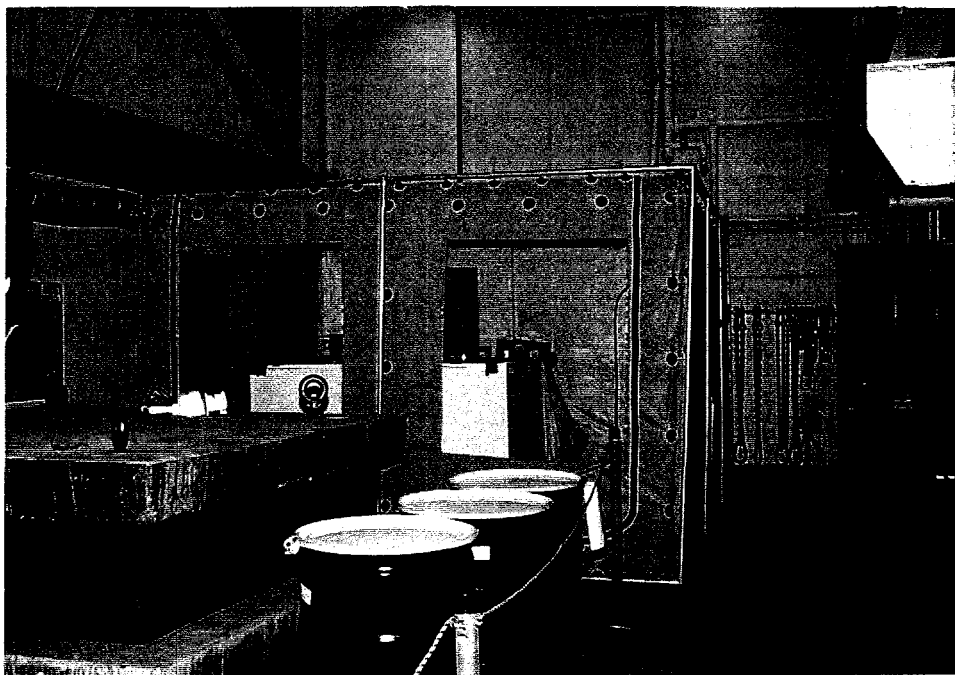
Figure 6.26 Containment Tent Over High-Dose Room Floor Opening (ANL Negative #22846K, Frame #10A)
