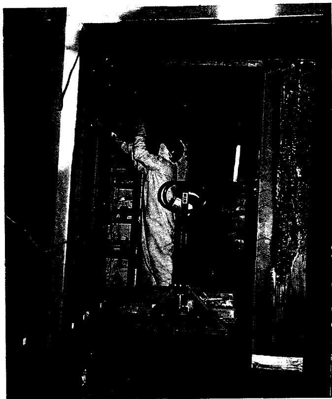
Figure 6.20 Technicians Removing Ceiling Lead from High-Dose Room (ANL Negative #22760K, Frame #10A)
