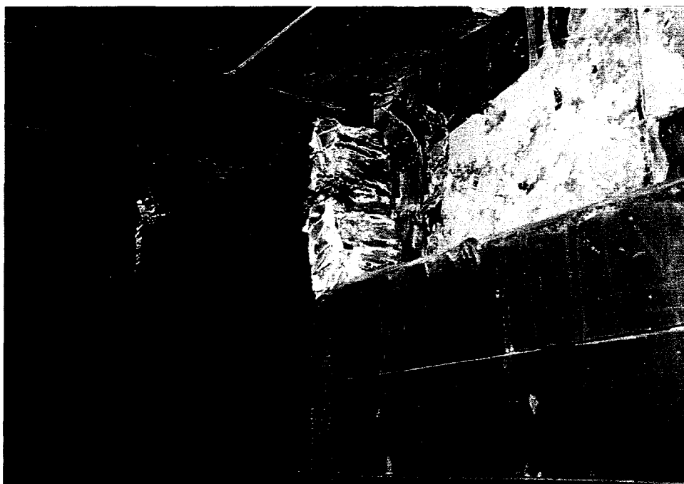
Figure 6.14 High-Dose Room Lead Wall Block Showing Full Depth Joint Weld (ANL Negative #22760K, Frame #12A)
