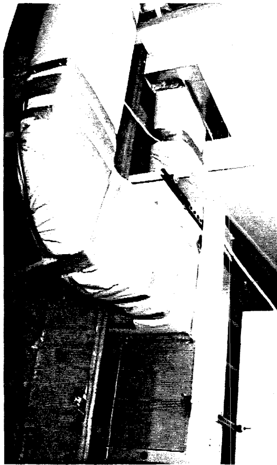
Figure 17. Heat pump unit suspended from garage ceiling.
