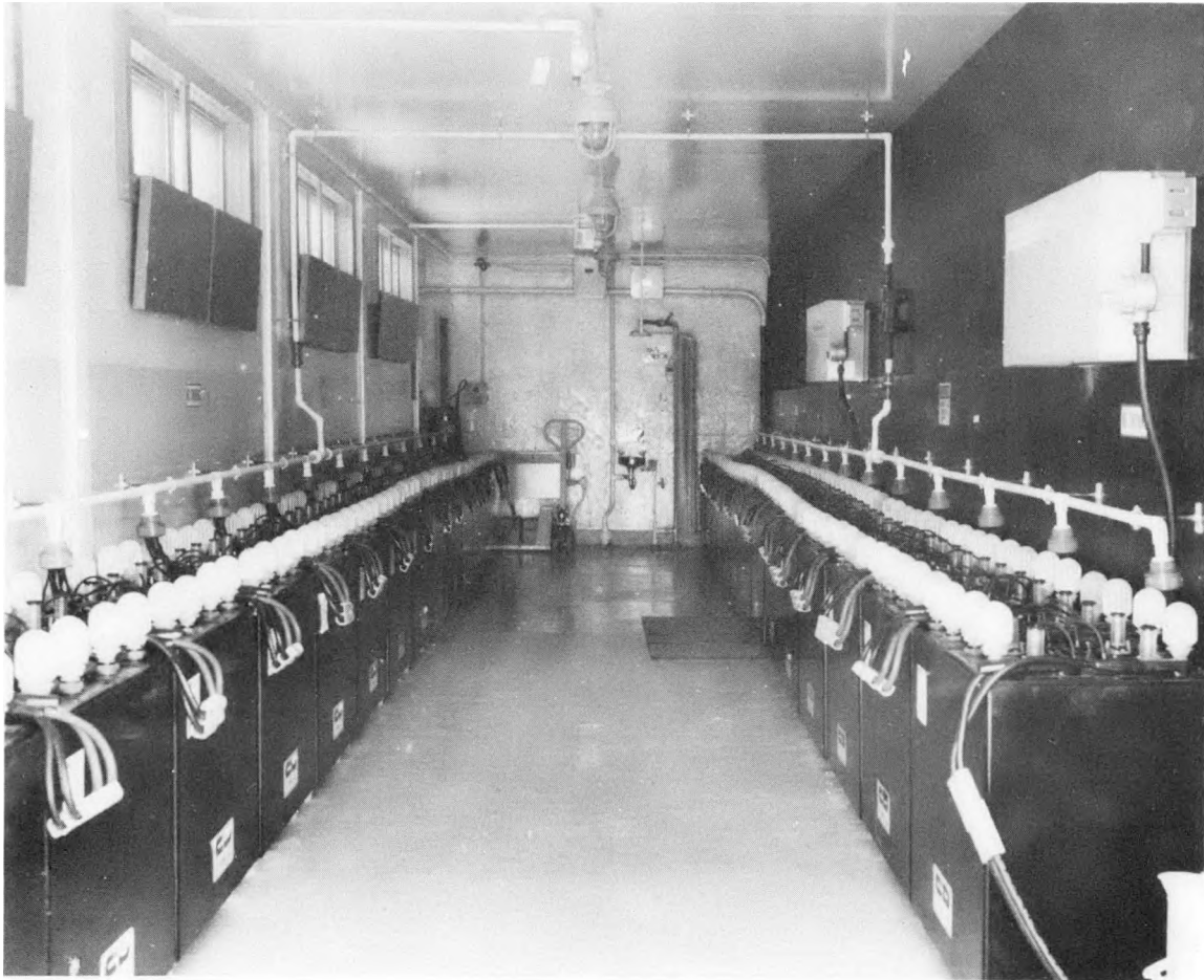
Fig. 7. PV building battery room.
