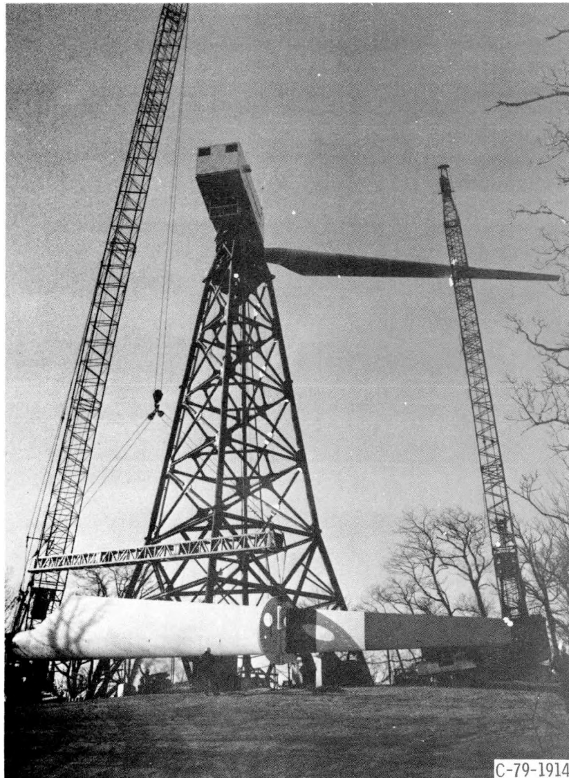
Figure 17. - Blade installation.
