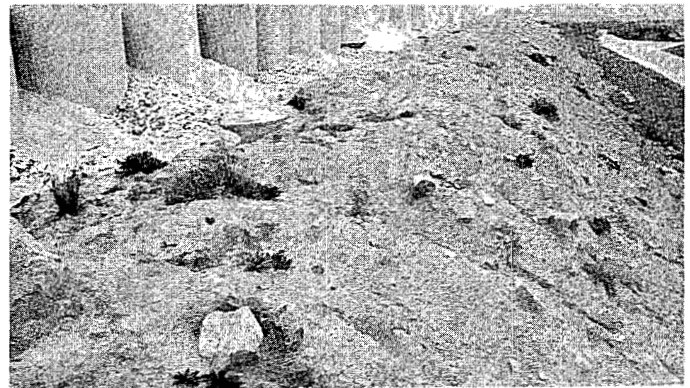
(2) The tumulus is built-up using a low permeability material to minimize infiltration.
