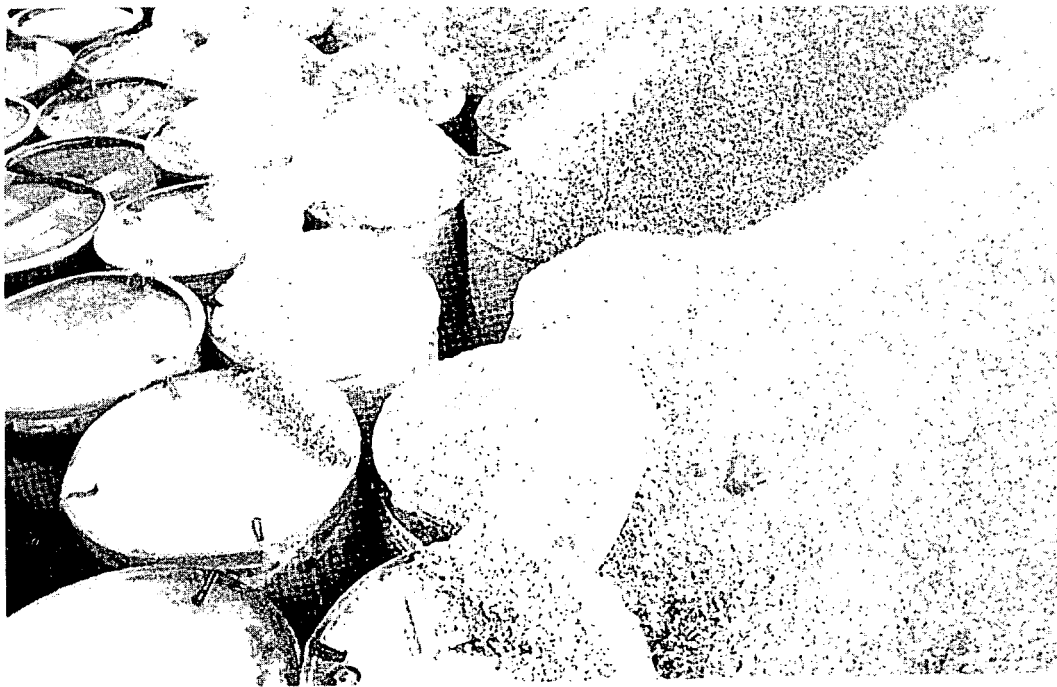
d. Backfilling of voids between waste packages
