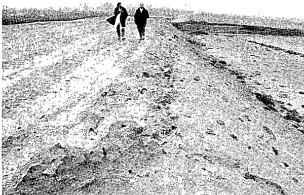
(3) Final shape of the tumulus is attained after the blocks and compartmentalized wastes have been completely covered.
