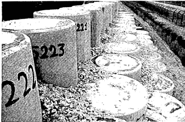
(1) Shape of the tumulus is initially formed by staking the waste packages around the perimeter in a stepped arrangement.
