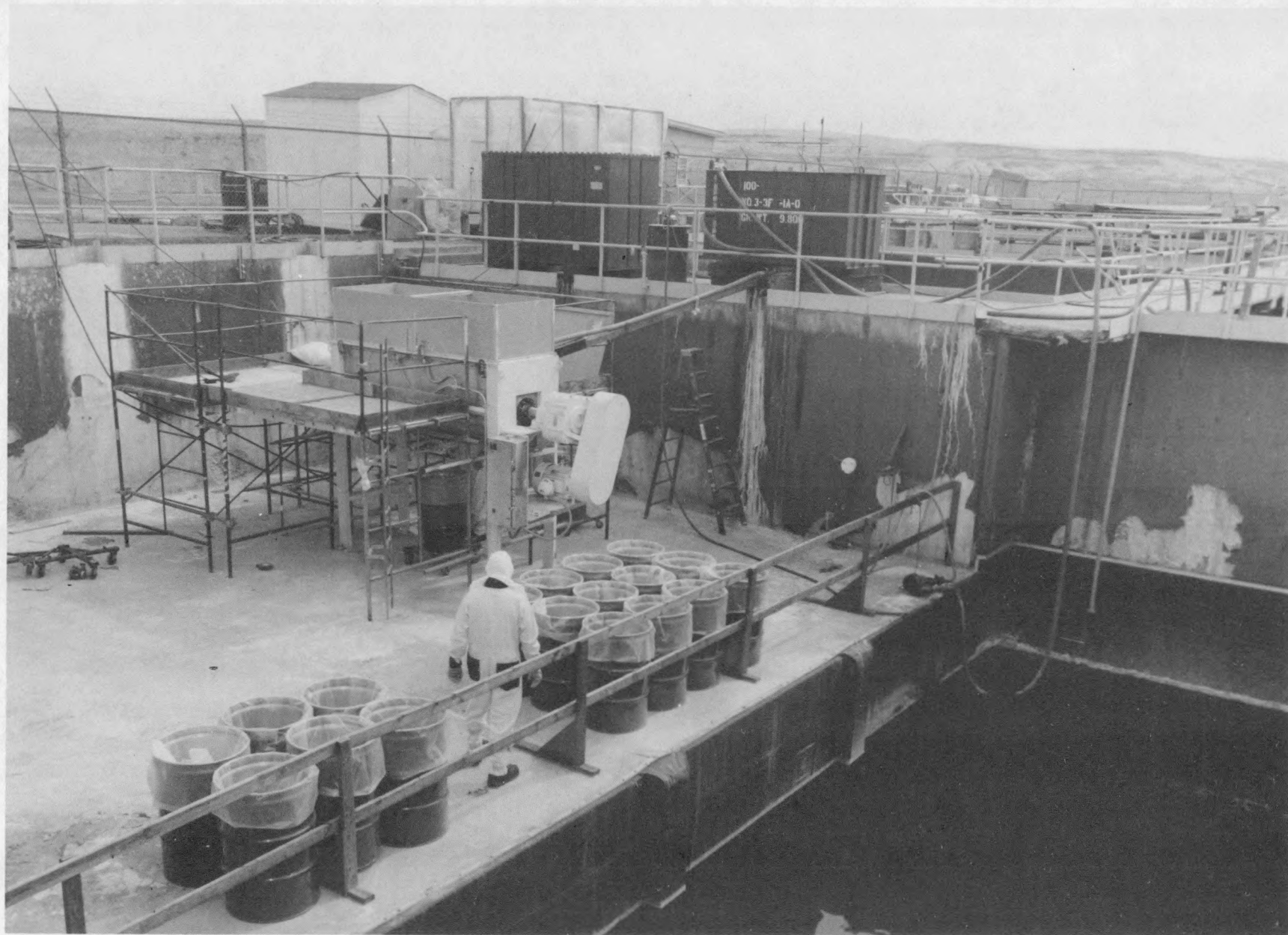
Figure 5. Solidification of Liquid Waste in 183-H Solar Evaporation Basins.
