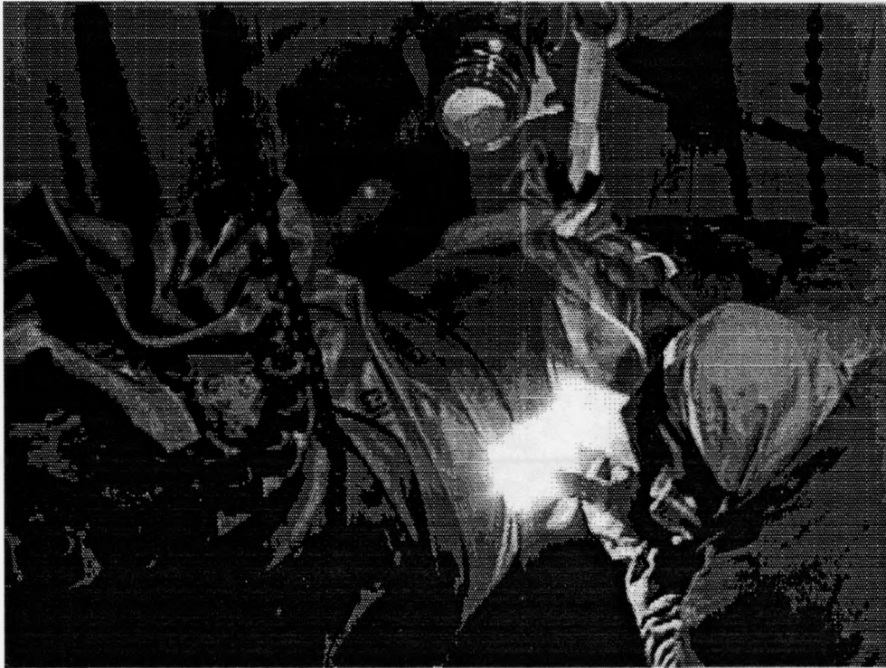
Photo 1. Plasma torch cutting of a reactor coolant pipe elbow (18-inch diameter, 1-1/2 inch wall thickness, stainless steel). Notice the portable air sampler positioned directly above the pipe. Average cutting time for this operation was about 30 minutes.
