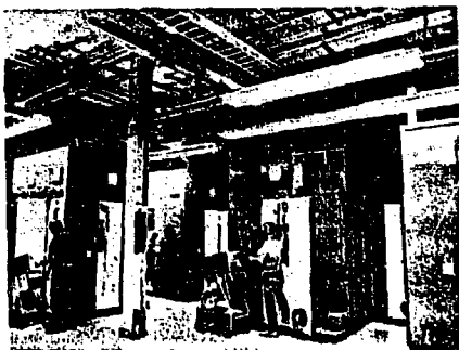
Fig. 9. The ECRH power supply system modulator/regulators manufactured by Universal Voltronics Corporation (UVC). Each of these cabinets have been recently installed on the first floor of Bldg. 431 and will provide regulated high voltage for a gyrotron positioned under the west MFTF-B vessel.
