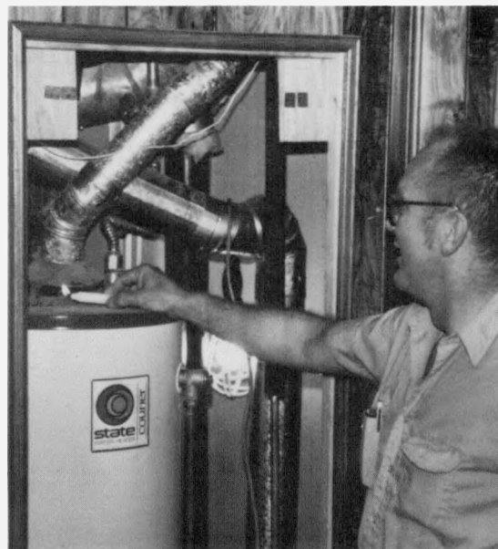
Figure 4-2. Checking to see if combustion appliances (natural draft-type) are susceptible to backdrafting of combustion gases (candle shows direction of air flow). (Photograph by Steve Andrews)
