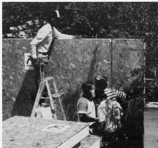
Figure 2-22. Foam-core panels (structural load bearing) being fit into place. (Photographs by Steve Andrews)
