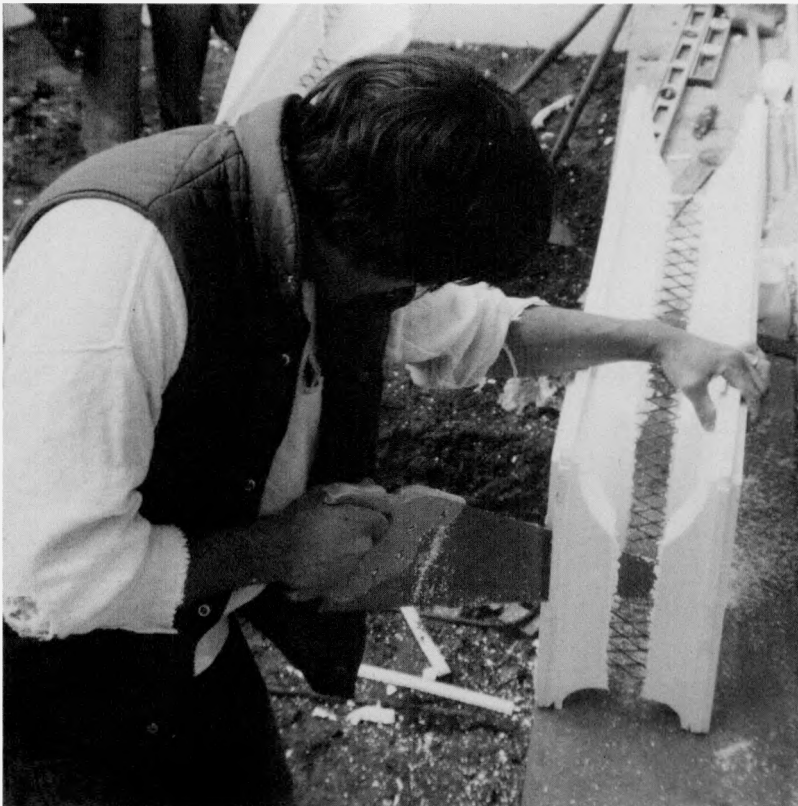
Figure 2-8. The Foam-Form® system: (A) Diagram of a Foam-Form block; (B) Cutting the foam-forming foundation; (C) Filling the block. (Source: Adapted from information supplied by Rocky Mountain Foam-Form.) (Photographs by Steve Andrews)
