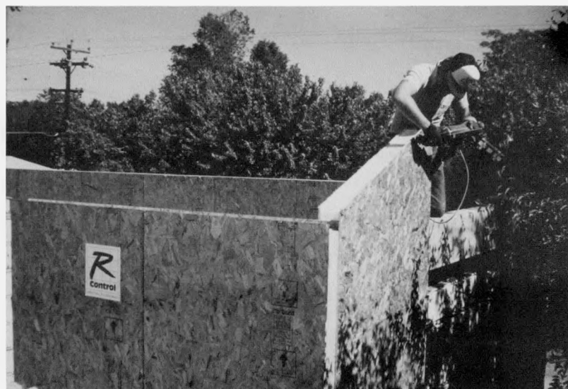
Figure 2-22. Foam-core panels (structural load bearing) being fit into place. (Photographs by Steve Andrews)
