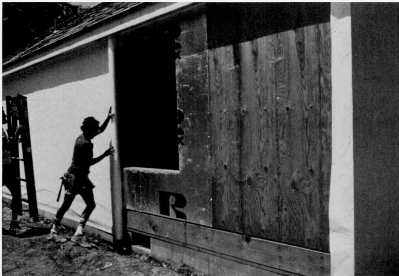
Figure 2-38. The interior air barrier film. (Source: Adapted from Nisson, J. D. Ned, and Gautum Dutt, 1985, The Superinsulated Home Book , New York: Wiley)
