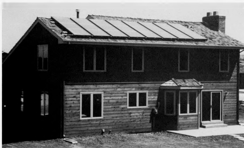
Figure 2-2. An example of a home with equivalent of 6% of its floor area in south-facing glass. (Photograph by Steve Andrews)
