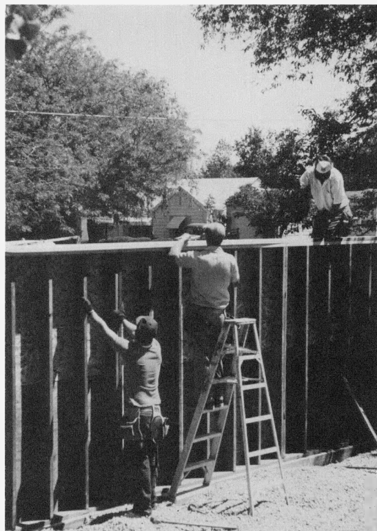
Figure 2-7. Permanent wood foundation that automatically includes space for insulation, eliminating some redundancy with conventional concrete foundations where interior insulation is desirable; walls for an average-sized home are placed in one morning. (Photograph by Steve Andrews)
