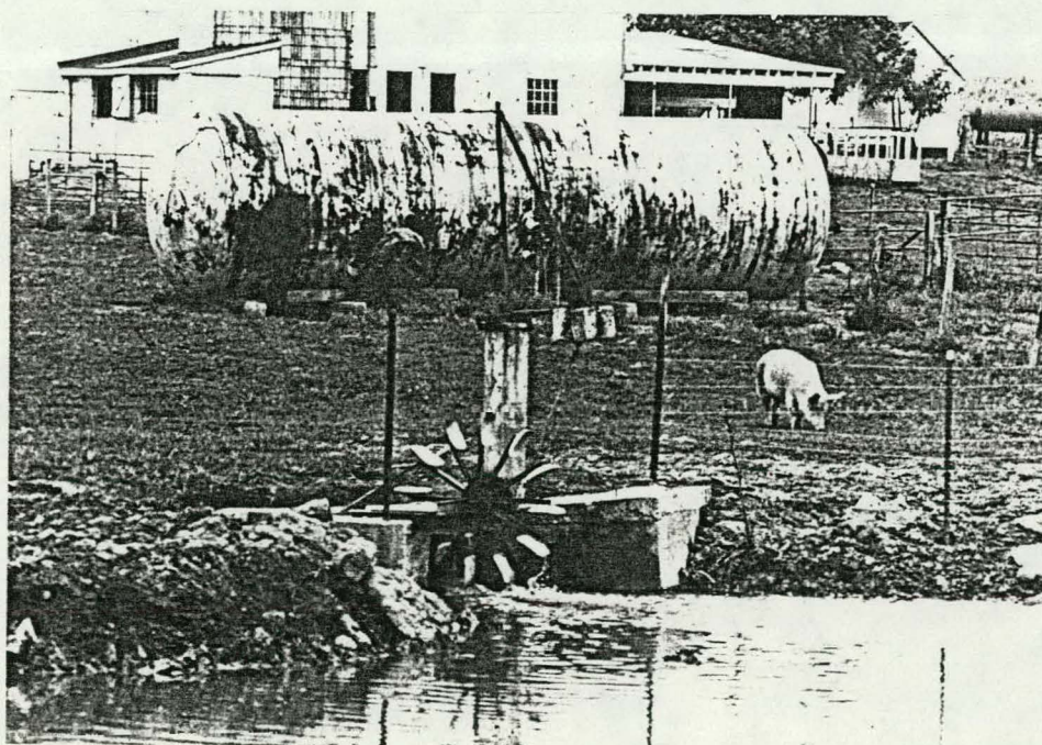
Figure 2. A "newer" type of Amish waterwheel. Lancaster County, Pennsylvania.
