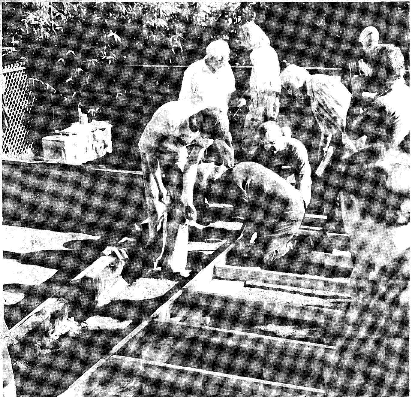
Framing up the front face of a solar greenhouse.
