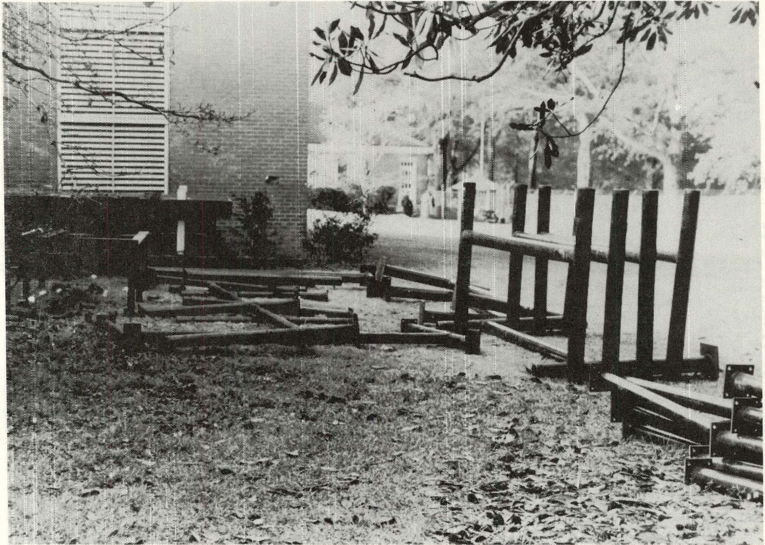
Figure 2-6. Collector Supports at Site, October 1977
