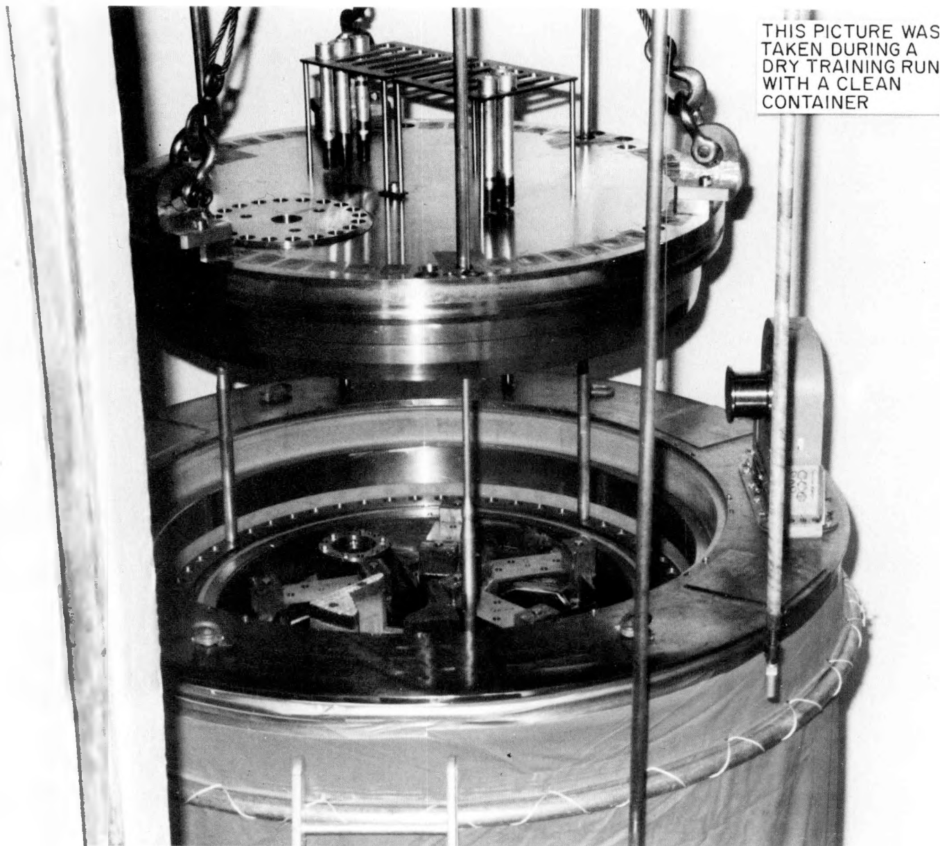
Figure 14. M-130 Closure Head Removal
