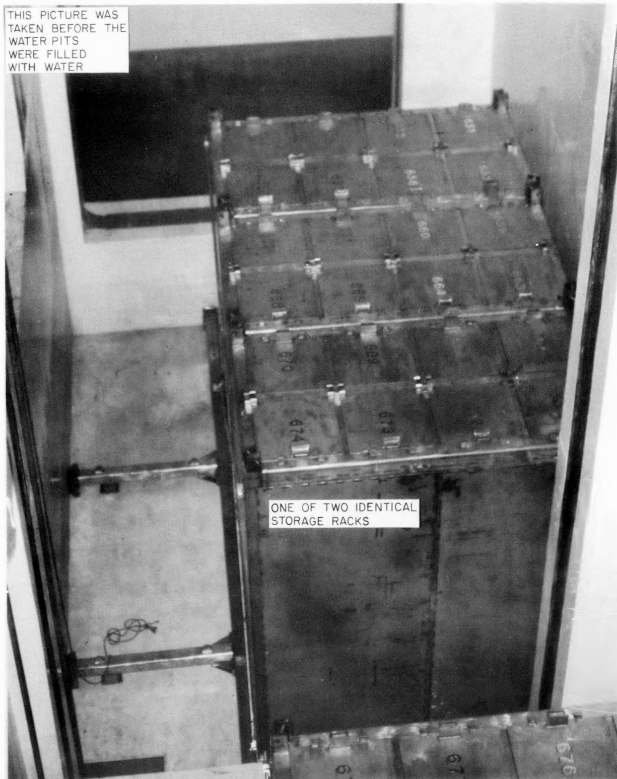
Figure 18. LWBR Fuel Storage Racks
