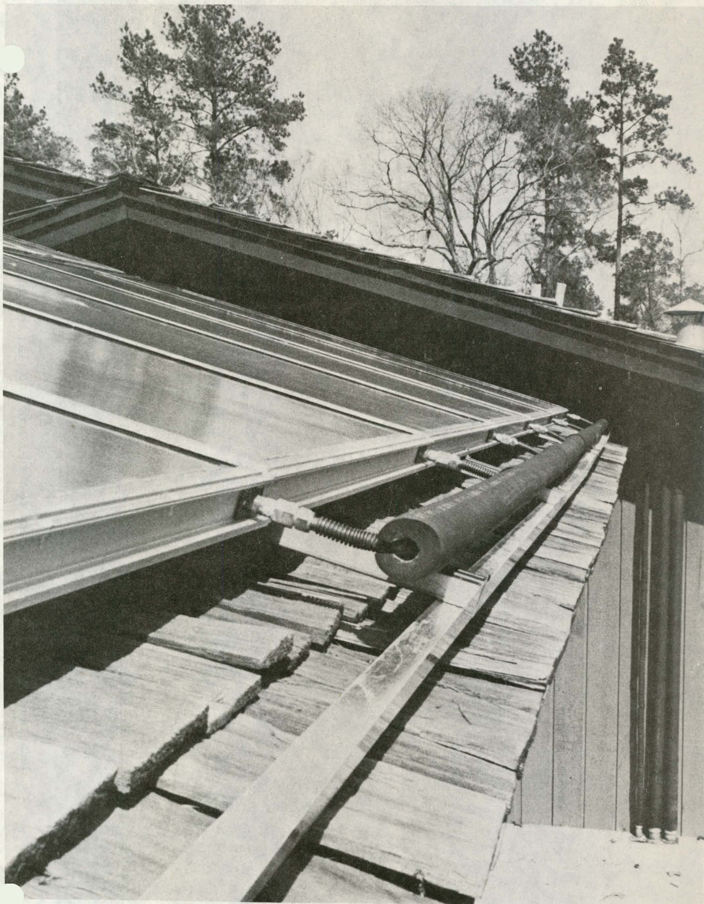
Typical installation of prefabricated manifolds.
