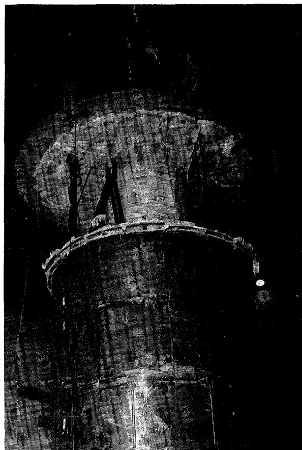
Figure 10.3 The Lower Portion of the Reactor Pressure Vessel at Marble Hill After the Thermal Annealing
