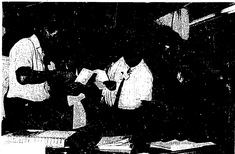
Merlyn Krick explains operation of active well coincidence counter to measure samples of highly enriched uranium.
