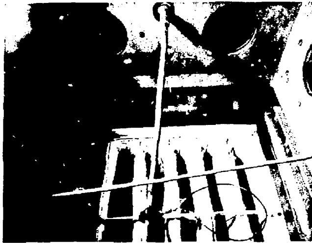
Fig. 111 Disposable prefilter installed in the filter housing.
