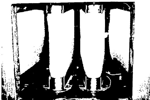
Fig. 135 Central filtering section of rolling electric prefilter.
