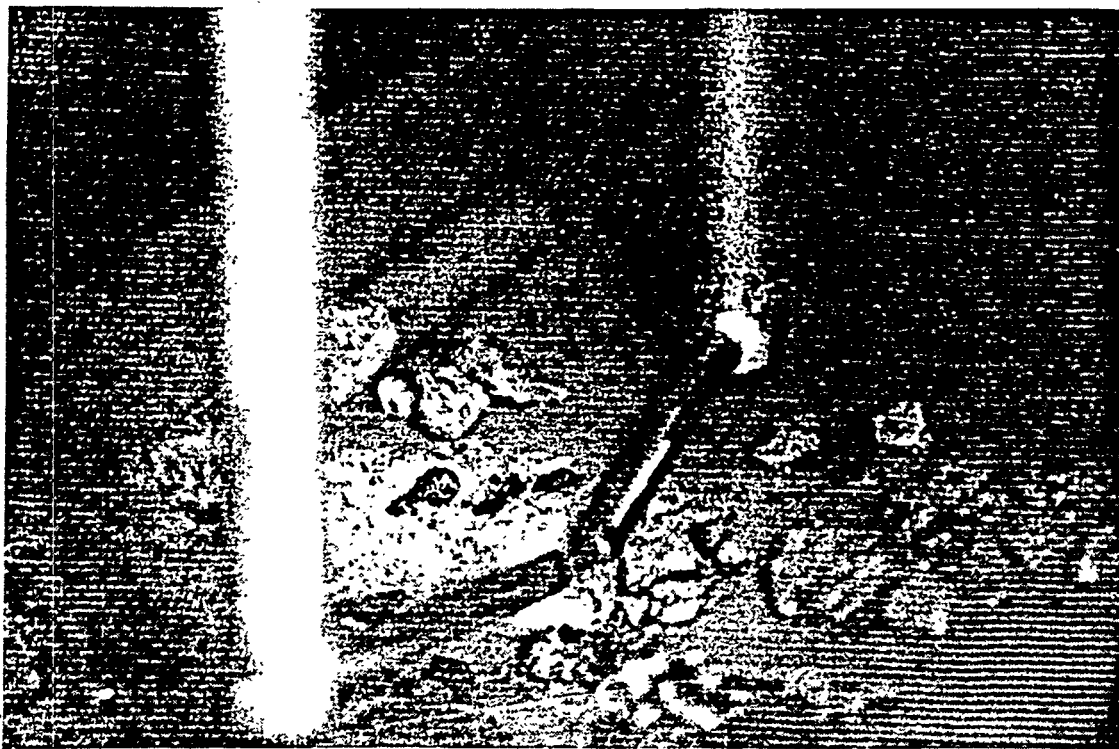
Figure 3-9 L-Shaped Electrode Configuration used to Prevent Misfire. Appearance of Scabbled Surfaces and Concrete Debris are also Shown
