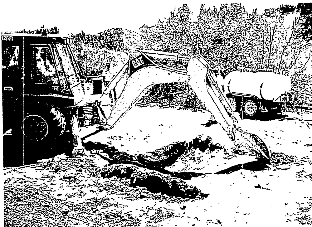
Figure 3.1.10 Backhoe Used to Remediate an Area Source
