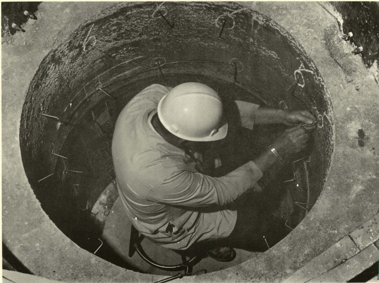
FIGURE 67. Installation of Anchor Extensions Prior to Casting the Dense Component.
