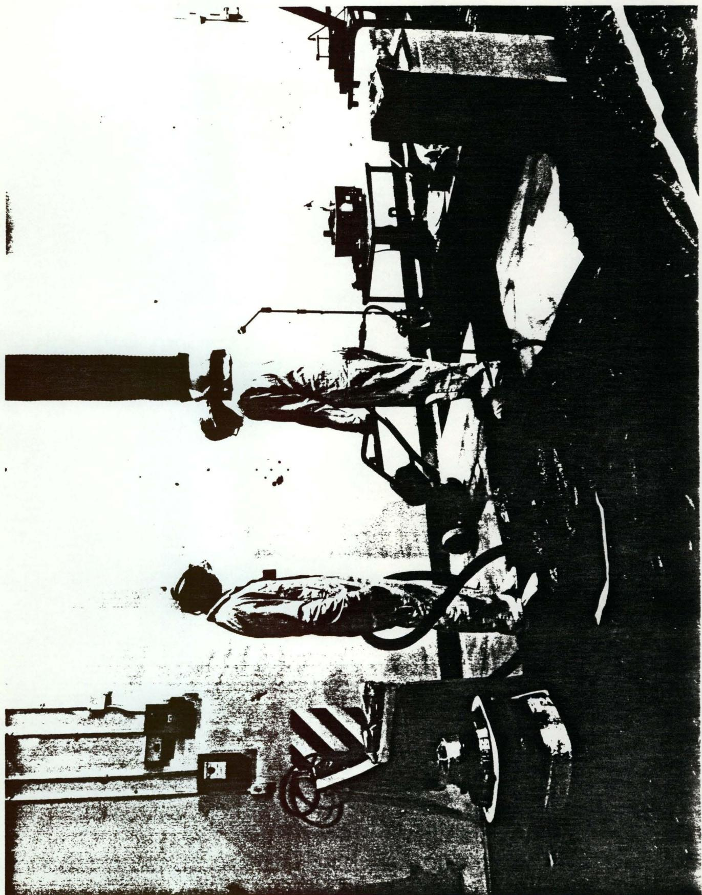
room air, assisting with the waste handling, etc. The two people need to alternate operating the scabbler to minimize fatigue. Experience indicates the confinement chamber is not necessary if surfaces are kept wet.
