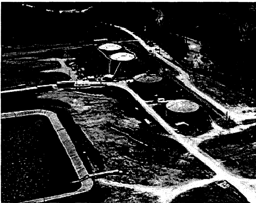
Figure 2-10 Waste Storage Tanks at Fernald
