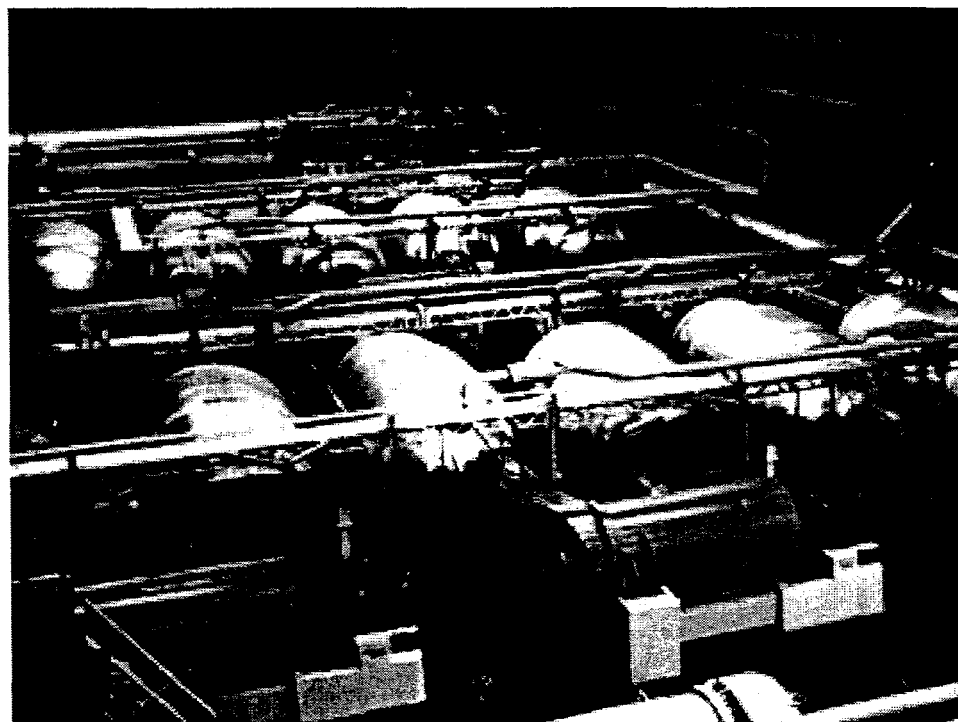
Figure 2-7. Thousands of diffusers and pumps will require removal at gaseous diffusion uranium enrichment plants.
