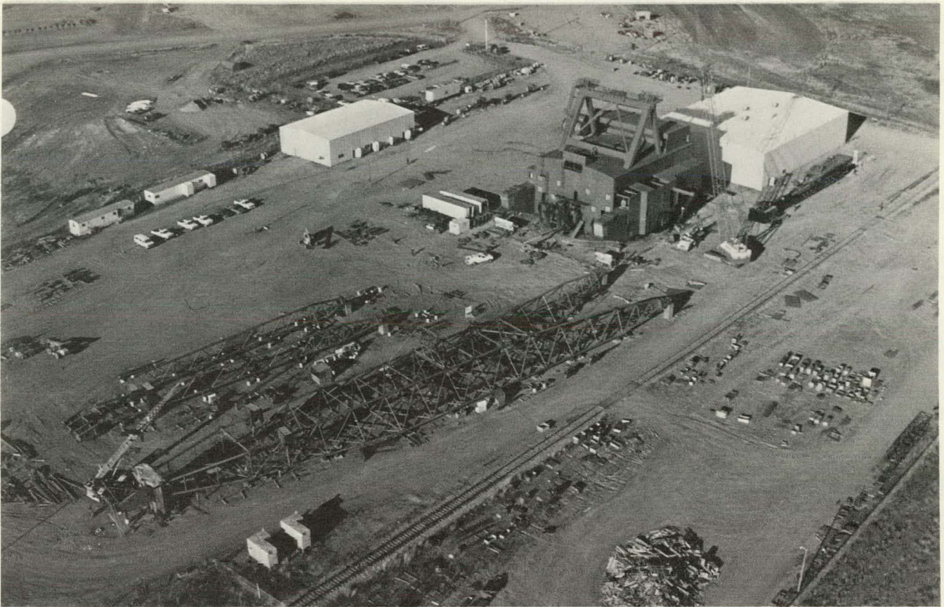
October 31, 1983—Code 2200—Dragline B. Erection—Erection Site
