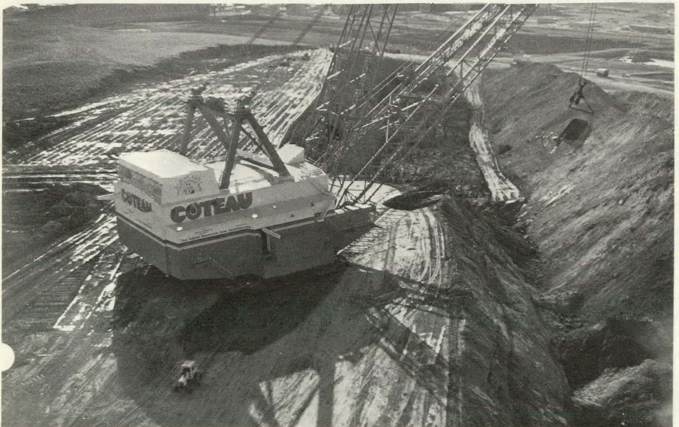
October 31, 1983—Dragline A—Removing Overburden
