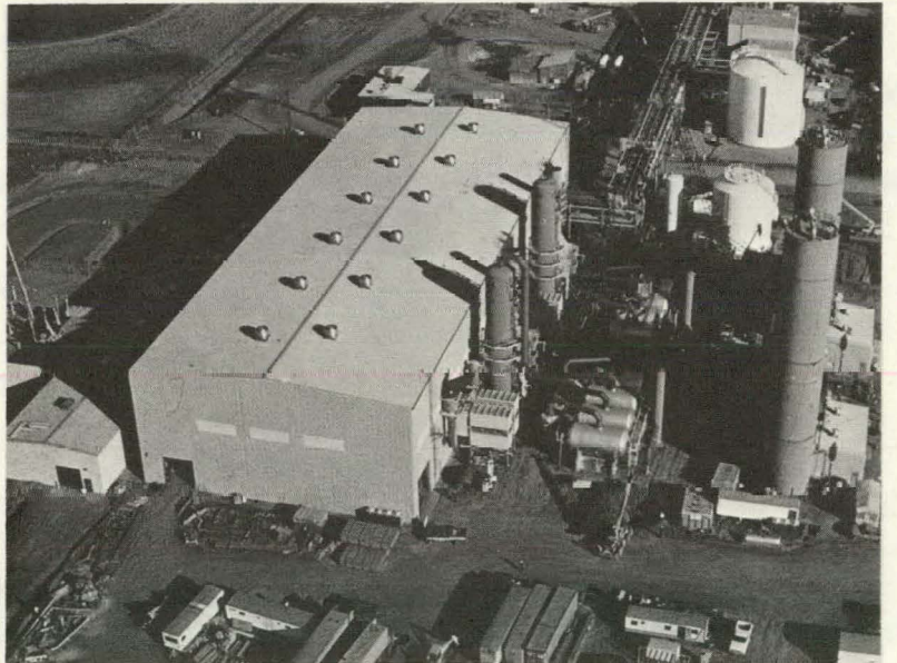
October 31, 1983—Area 3000—Oxygen Plant and Main Electrical Substation—Looking East
