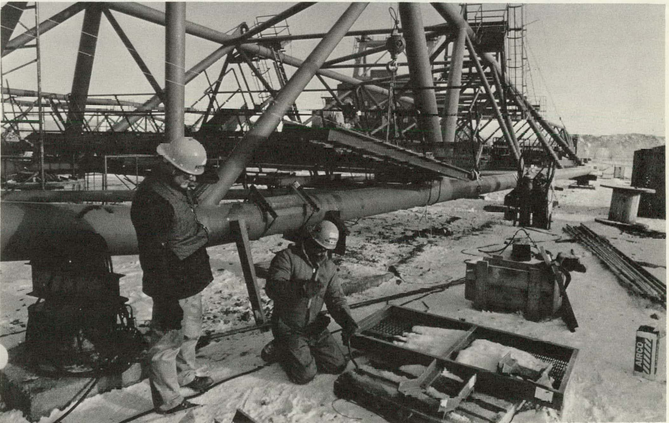
December 6, 1983—Code 2200—Dragline B Boom Fabrication and Welding
