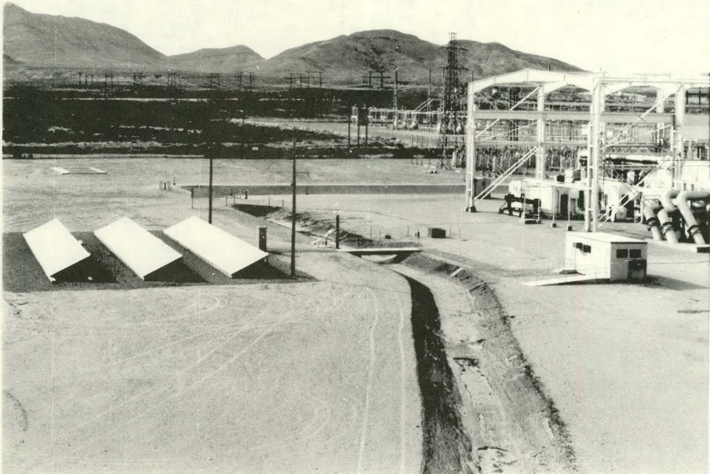
Figure 2. Photovoltaic Array, Newman Power Station
