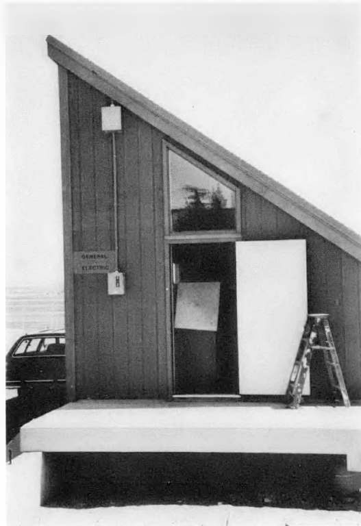
Figure 2-31. DC Power Drop Line
