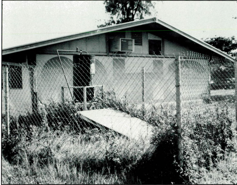
(Solar water heating system at the Marianas High School - not operating - 1986.)
