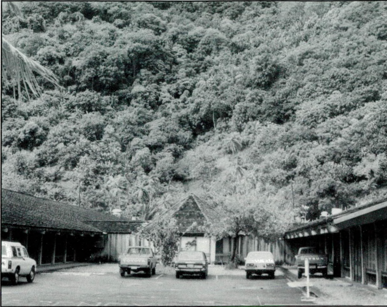
(Back of the Hospital where the solar air conditioner is located - 1980.)
