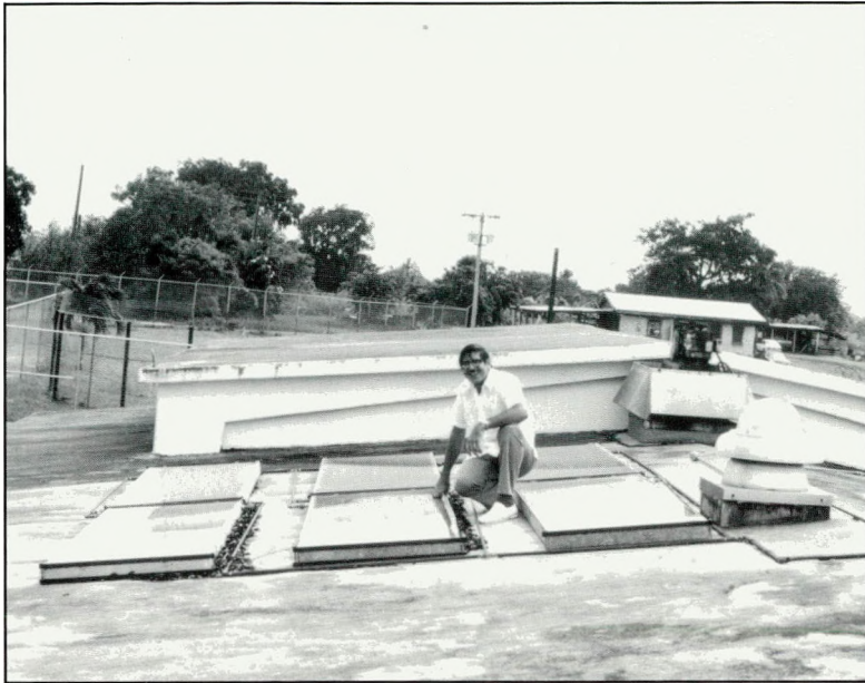
(Frank Jaquette inspecting his solar collectors on a youth detention home - 1981.)
