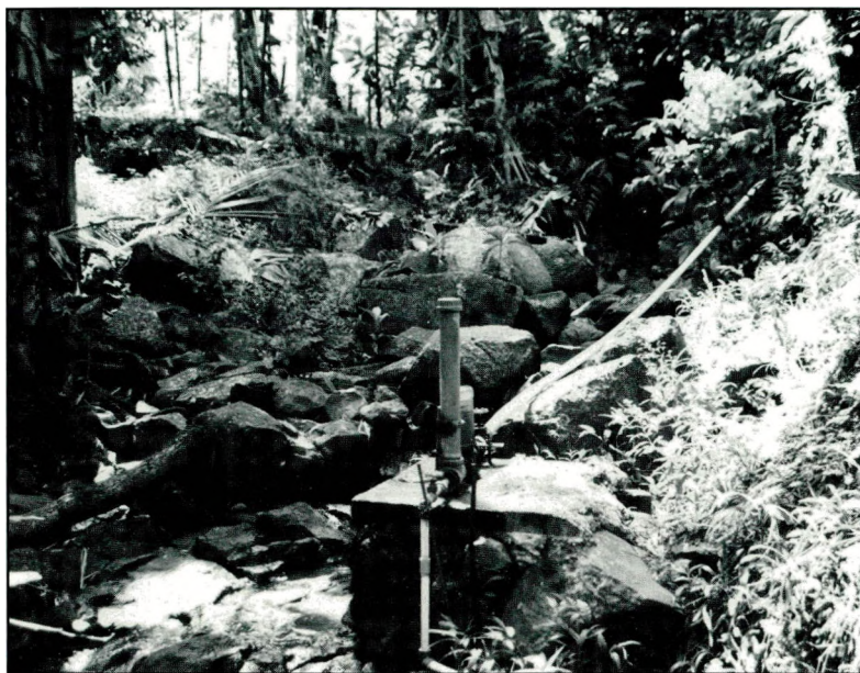
(Ram water pump near Ipwal Village - 1986.)
