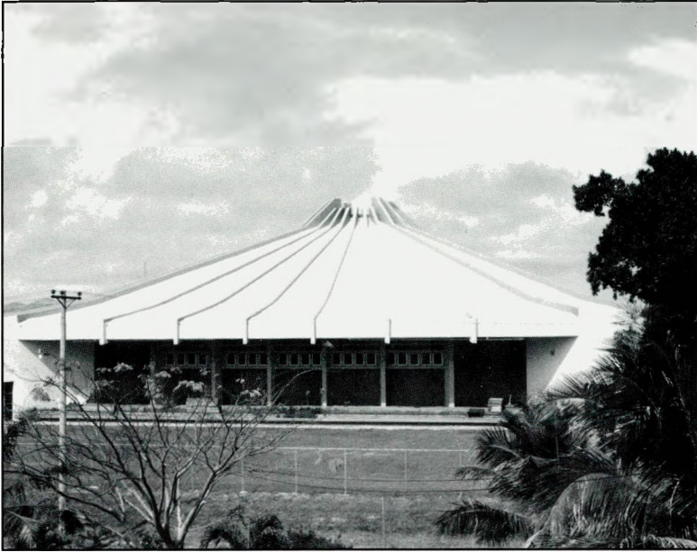
(University of Guam gymnasium - solar collector is on the far left - 1986.)
