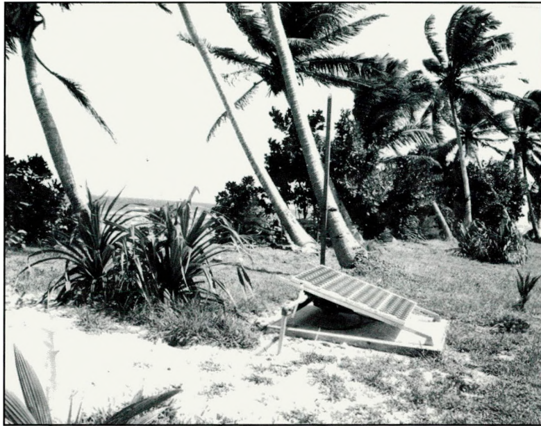
(Photovoltaic pumping system on Majuro - 1986.)
