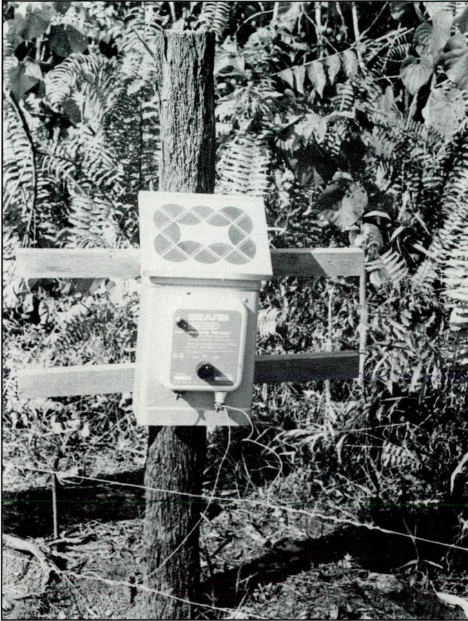
(Photovoltaic system for powering the electric fence at PATS - 1983.)
