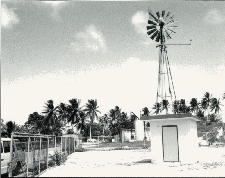
(The pump house and Dempster windmill - Majuro - 1986.)
