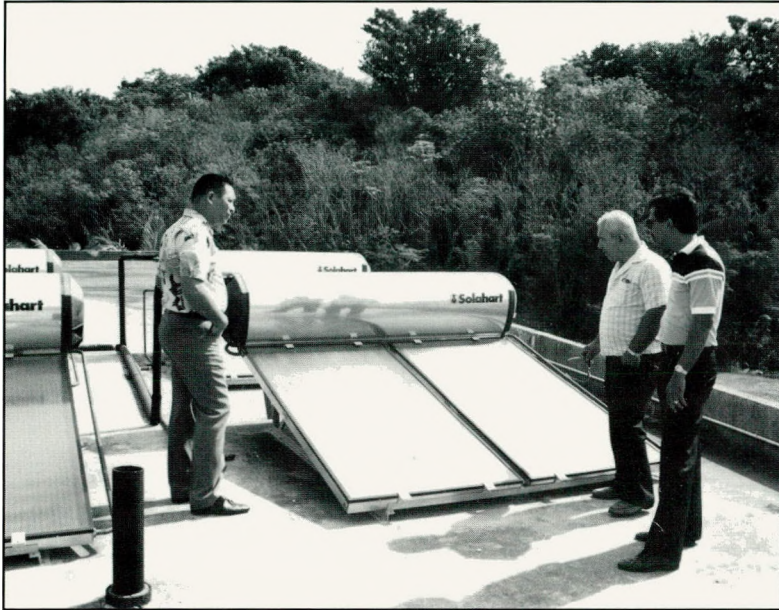
(SolaHart collectors at a University of Guam dormitory - 1986.)
