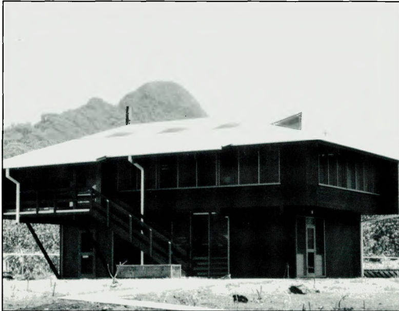
(Front view of the American Samoa Territorial Energy House - 1982.)
