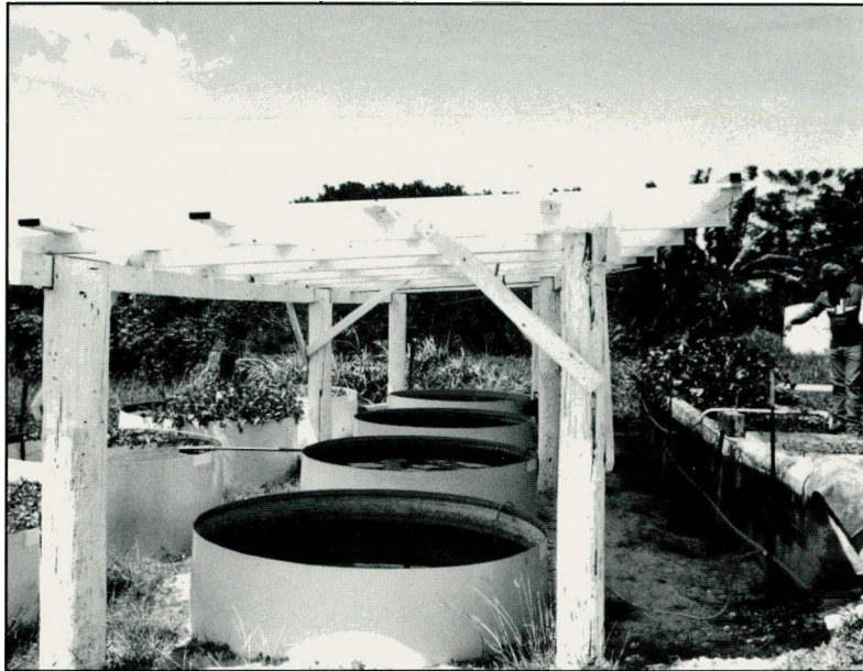
(Digester and aquaculture ponds at the integrated digester plant - As Lito Agriculture Station - 1985.)
