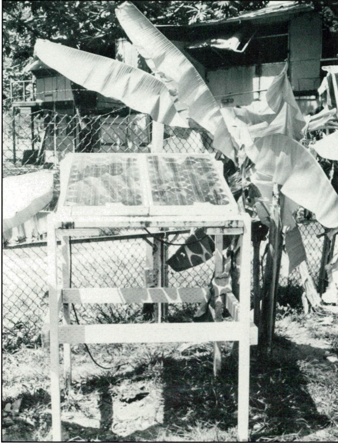
(Photovoltaic demonstration system at the South Pacific Mobile Training Unit - Majuro Atoll - 1982.)
