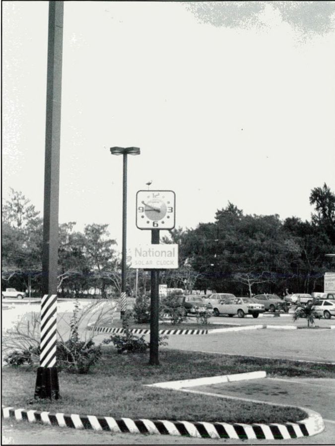
(Photovoltaic panel above the clock, Susupe Shopping Center - 1982.)
