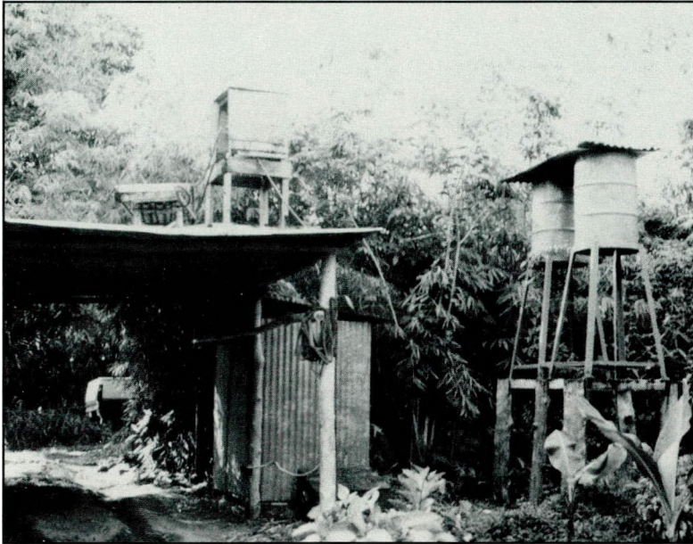
(Water storage and heating systems - 1980.)
