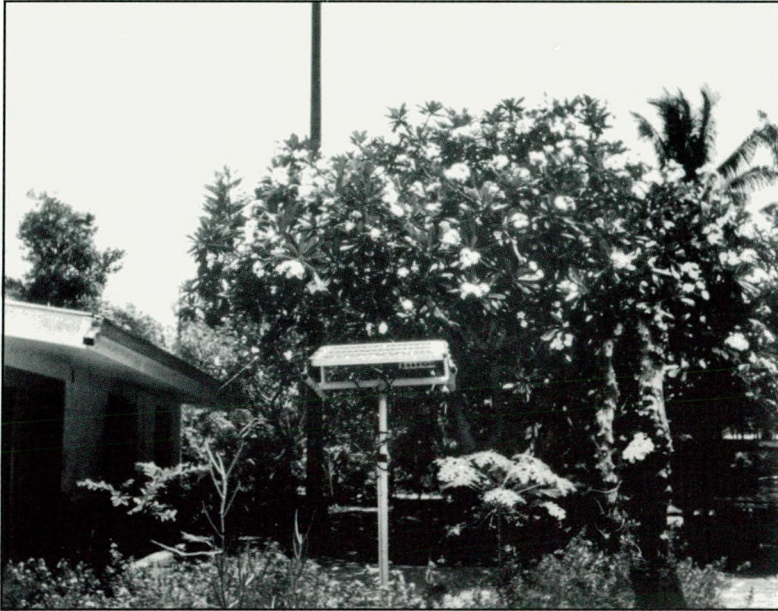
(Part of the photovoltaic powered communication system - Palau - 1985.)
