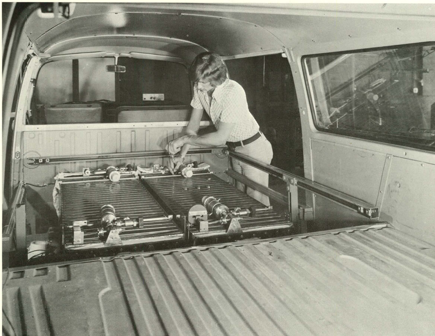
Fig. III-11. Mark IA Modules Installed in Volkswagen Transporter Van. ANL Neg. No. 308-79-319.
