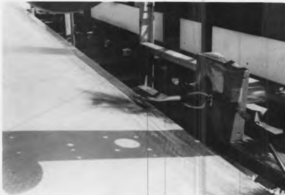
(a) Post-test damage.
