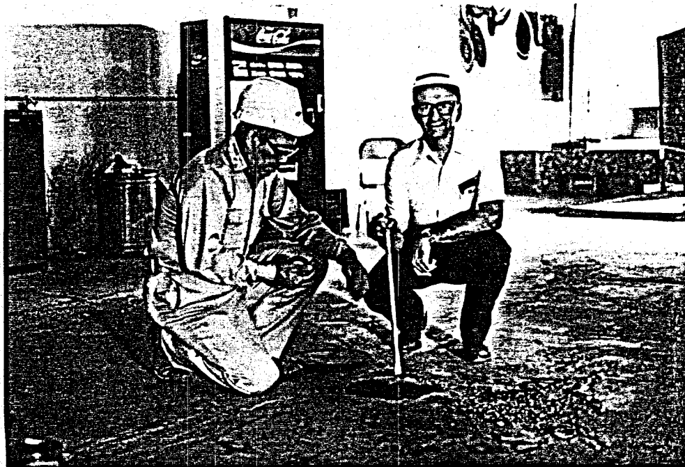
Figure 7. Mr. Drunzer and Alfred Armijo inspecting the sump in the Teen Center. The water level is about 2 1/2 feet below the surface.
