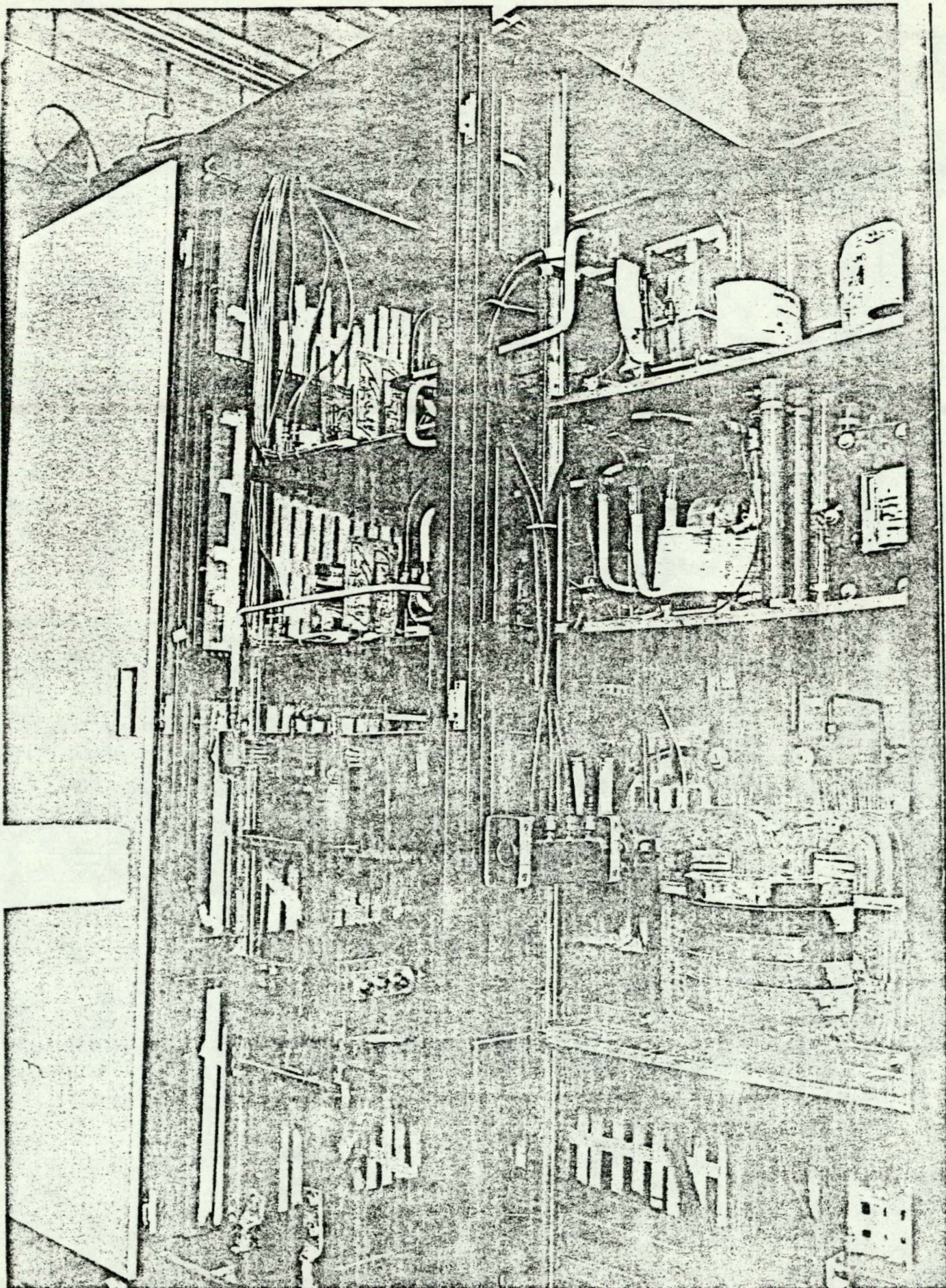
SWITCH ASSEMBLY NSLS UV DIPOLE POWER SOURCE FIGURE 5
