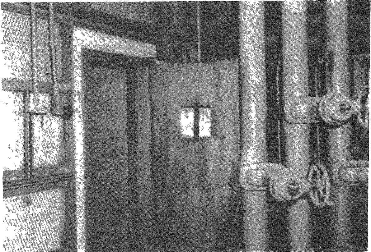
Figure 3. Enclosed stairwell door on the 305-foot elevation indicating overpressure damage.
