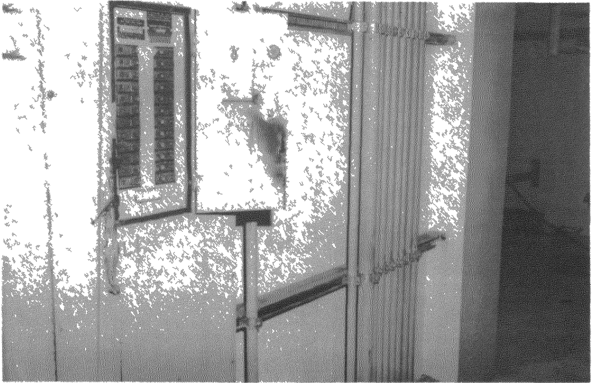
Figure 22. Charring and melted door seal material on electrical panel in southeast area of the 347-foot elevation.
