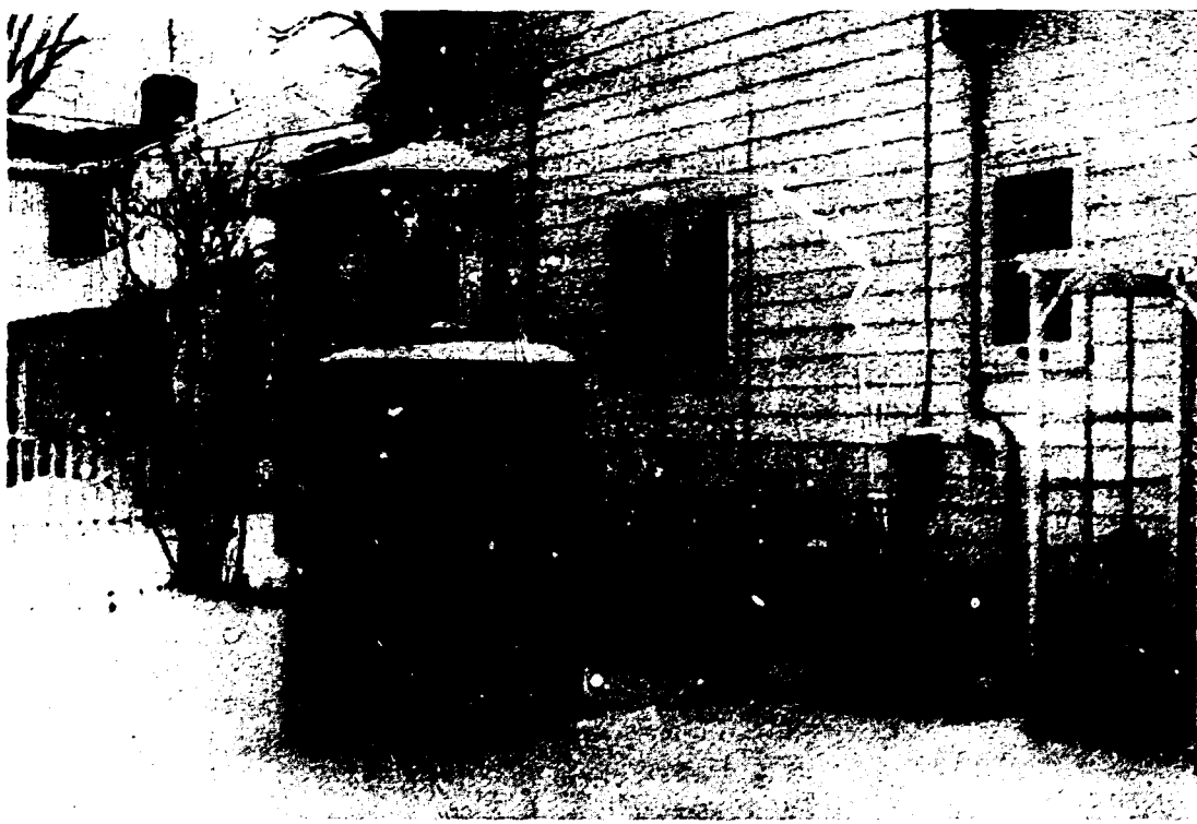
Fig. 6.1. Field-trial installation of an organic working-fluid residential absorption heat pump developed by Allied Corporation and cofunded by Gas Research Institute and DOE.
