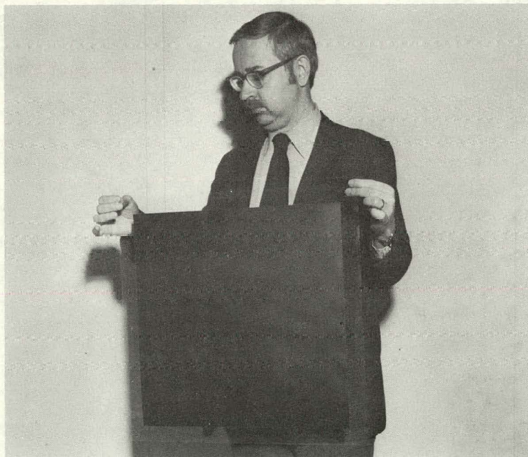
Figure 2.3. 2-1/2 Ft 2 membrane and electrode assembly
