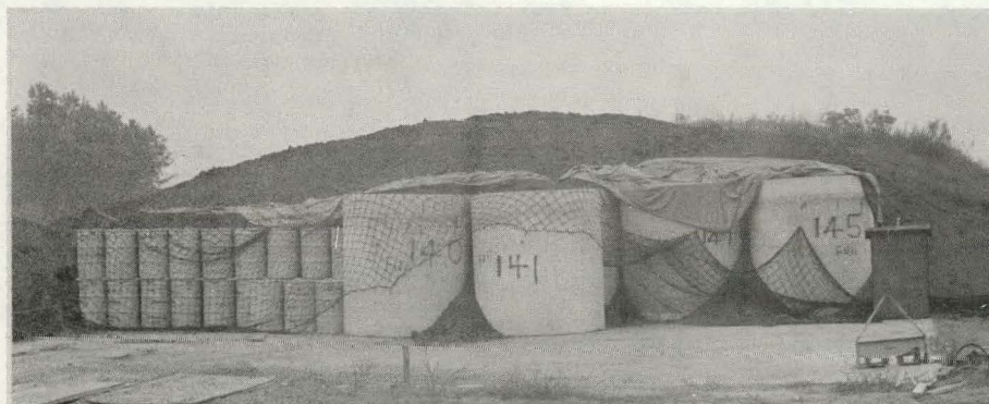
FIGURE 2. Retrievable Storage of TRU Solid Waste at the Savannah River Plant
