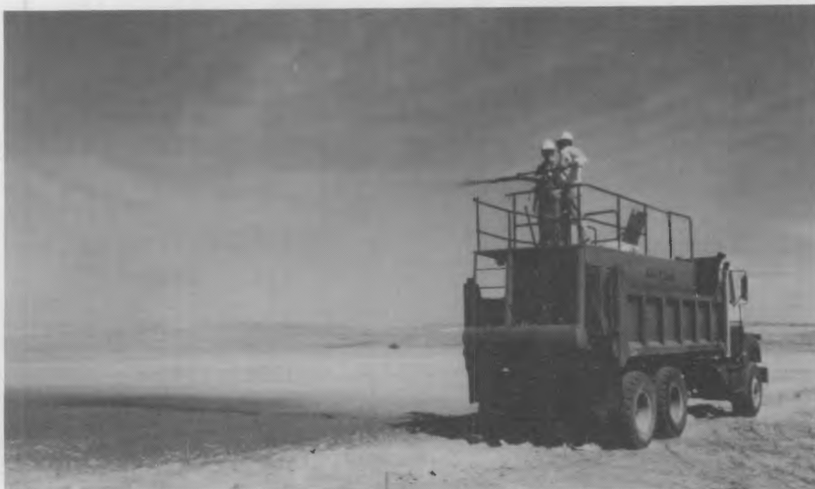
FIGURE 14. Application of Hydro Mulch (wood fiber/water slurry) with Hydroseeder
