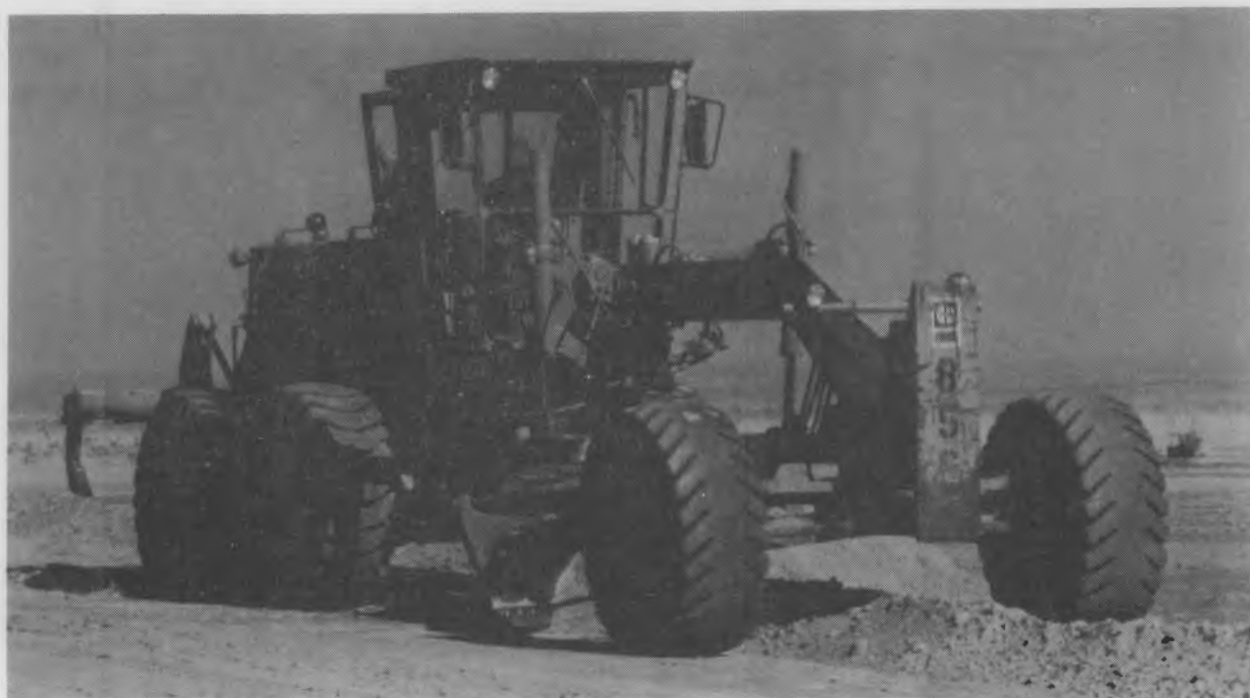
FIGURE 8. Grader Removing Treated Surface Tailings from Test Plot Area
