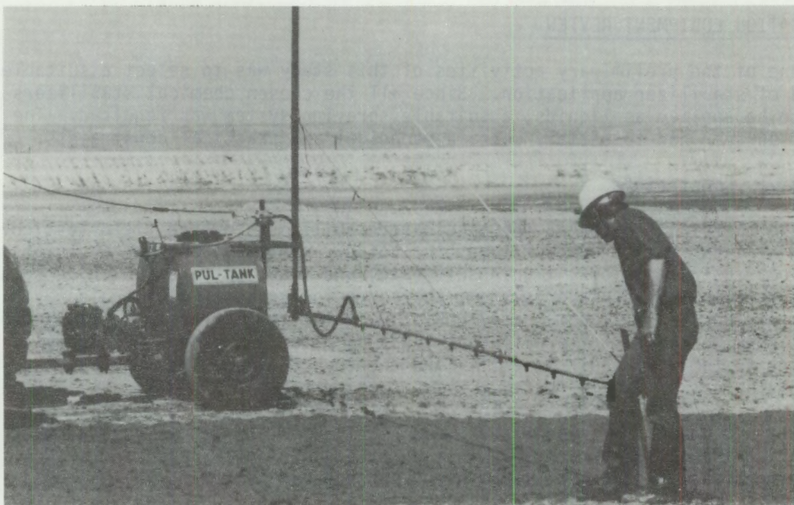
FIGURE 5. Application of Chemical Stabilizers with a Small Field Sprayer
