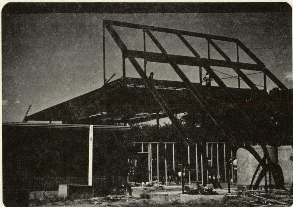
Steel Framing for Collector Roofing and Structure
