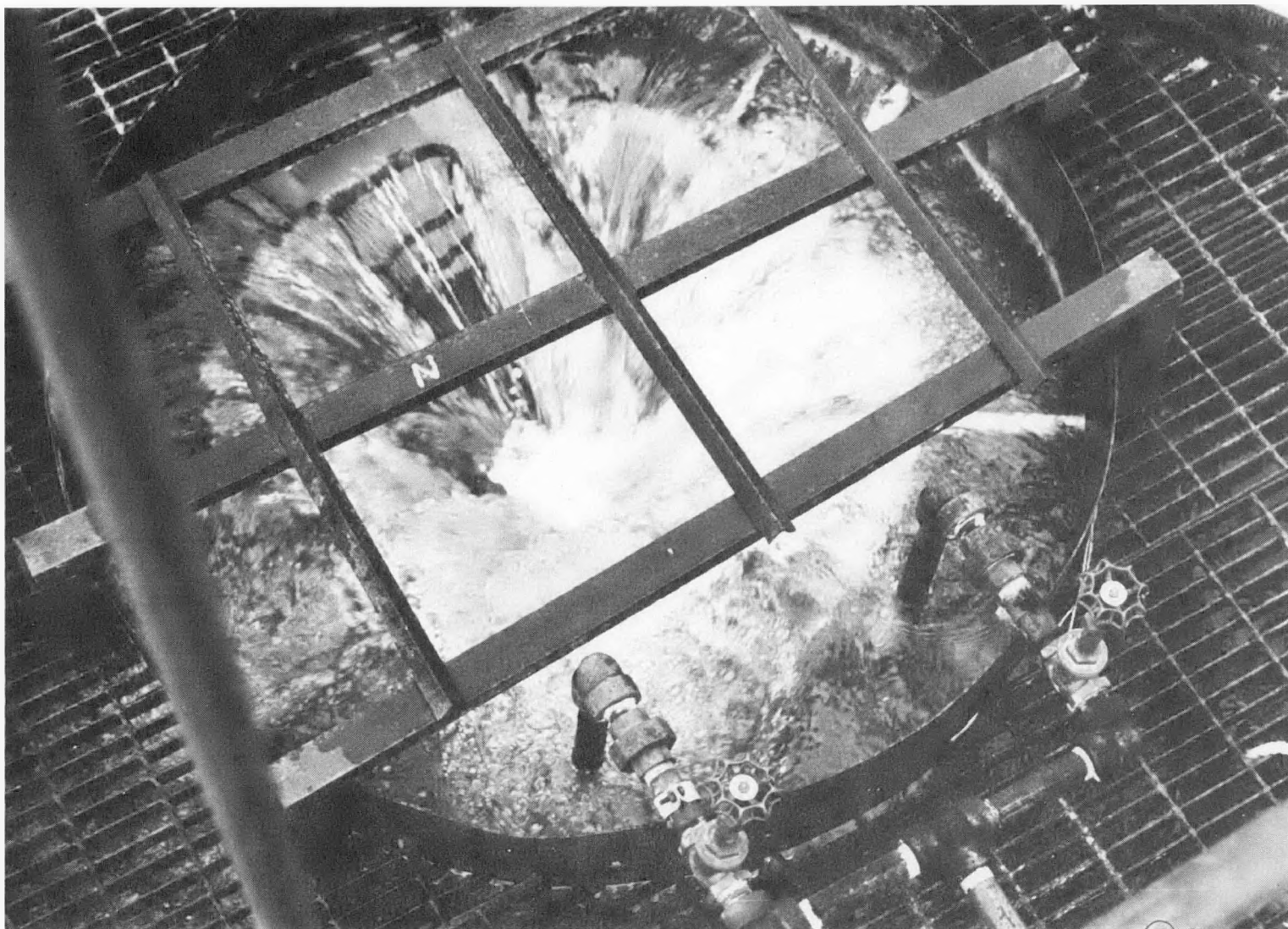
Figure 6-27. Treatment of Ash Pond Effluent With Carbon Dioxide, Rush Island
