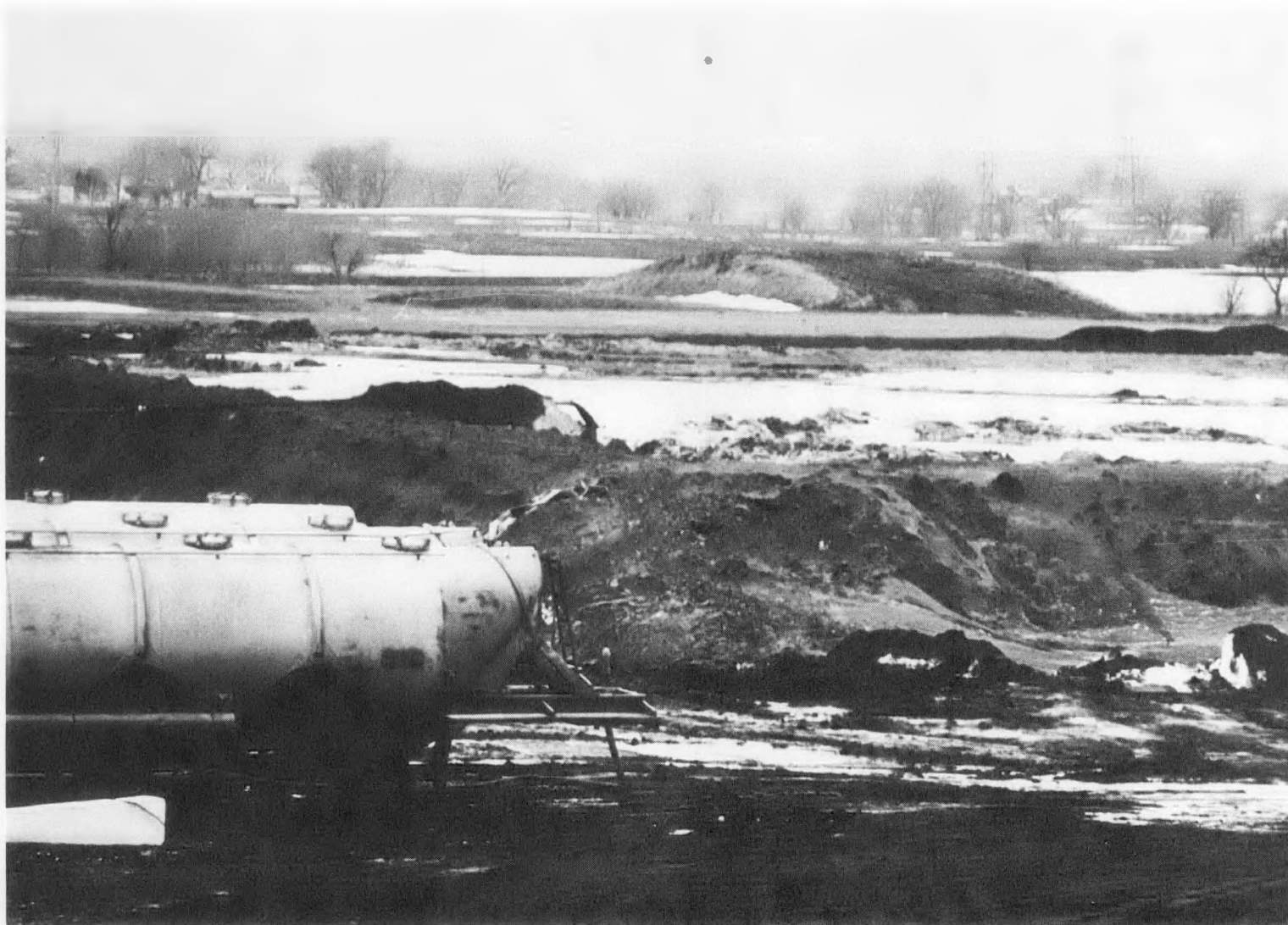
Figure 6-43. Ash Disposal Area, Waukegan
