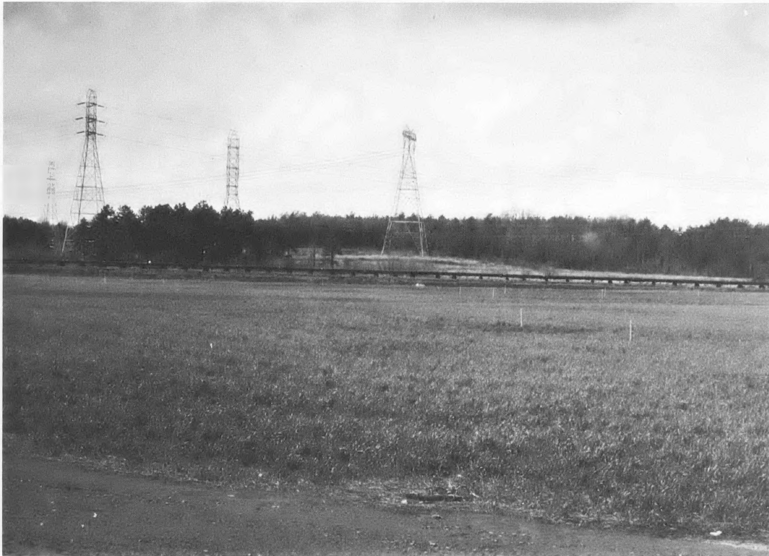
Figure 6-5. Revegetated Pond Areas at Allen Station
