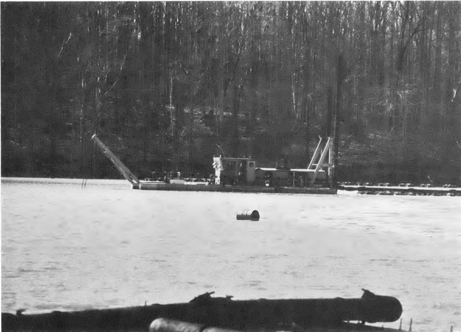
Figure 6-39. Ash Dredge, Marshall
