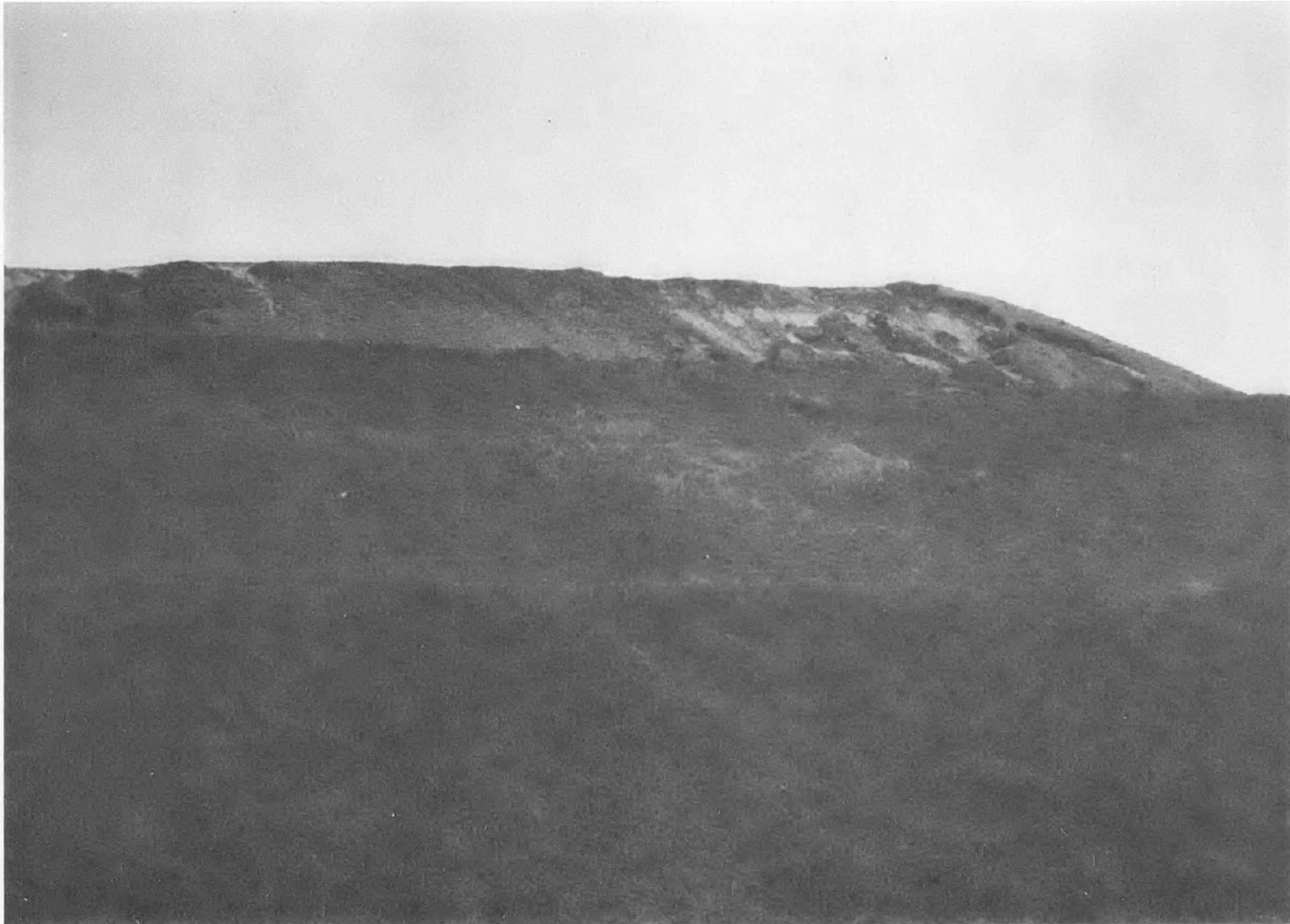
Figure 6-13. Ash Embankment, Keystone Station
