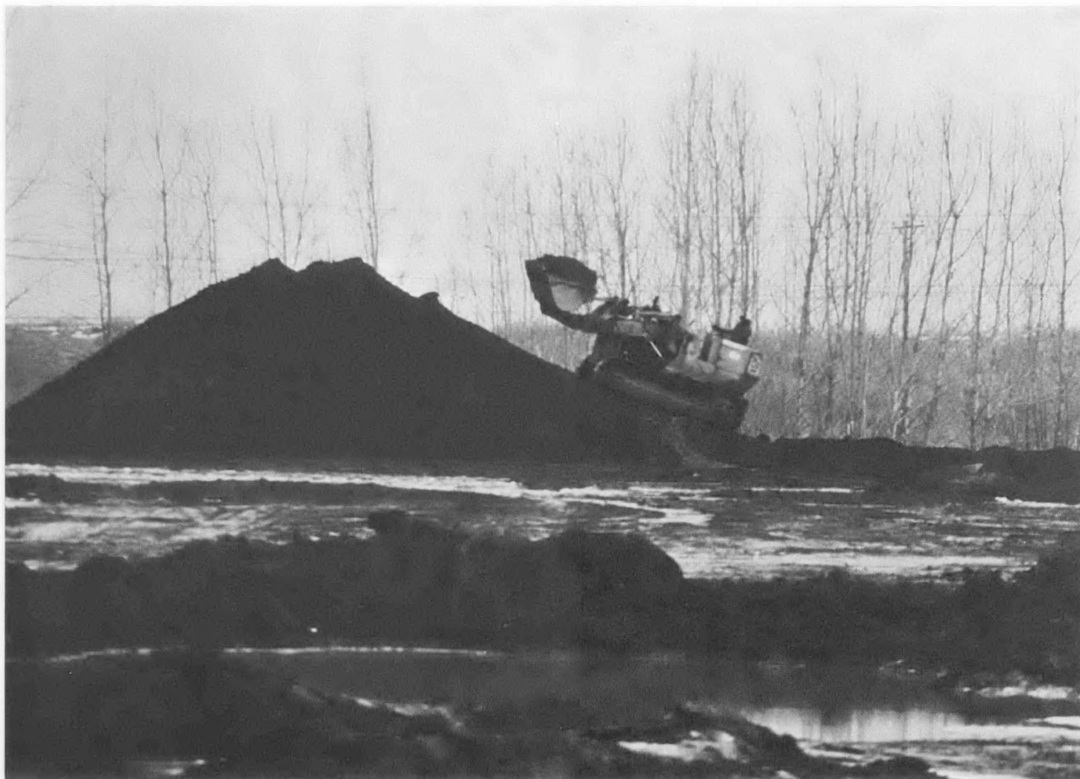
Figure 6-25. Bottom Ash Excavation, Labadie
