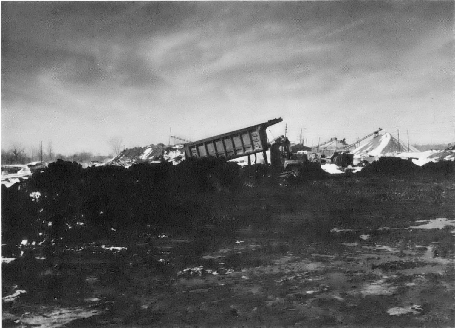
Figure 6-41. Ash Placement, Front Street
