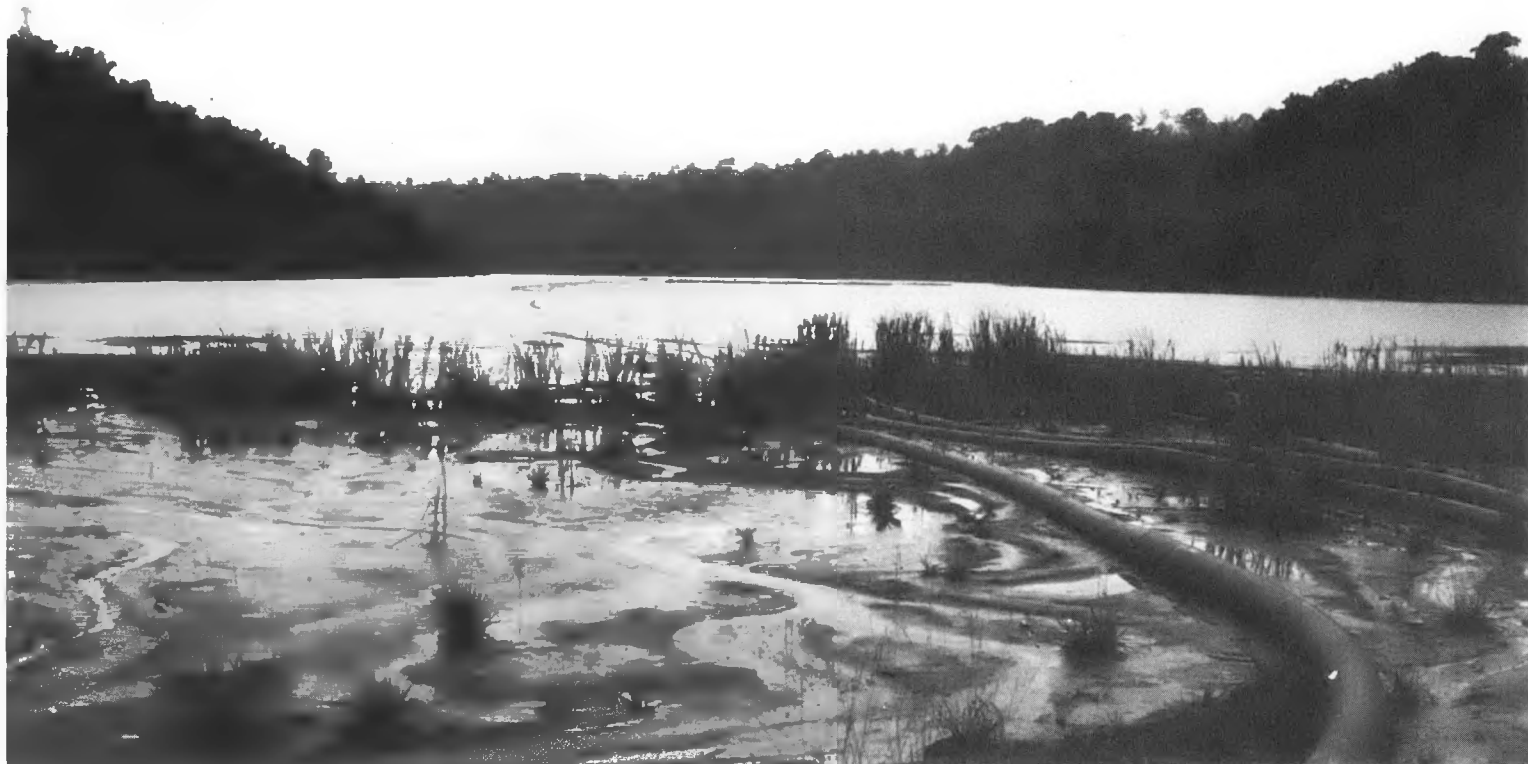
Figure 6-38. Floating Slurry Lines, Clifty Creek
