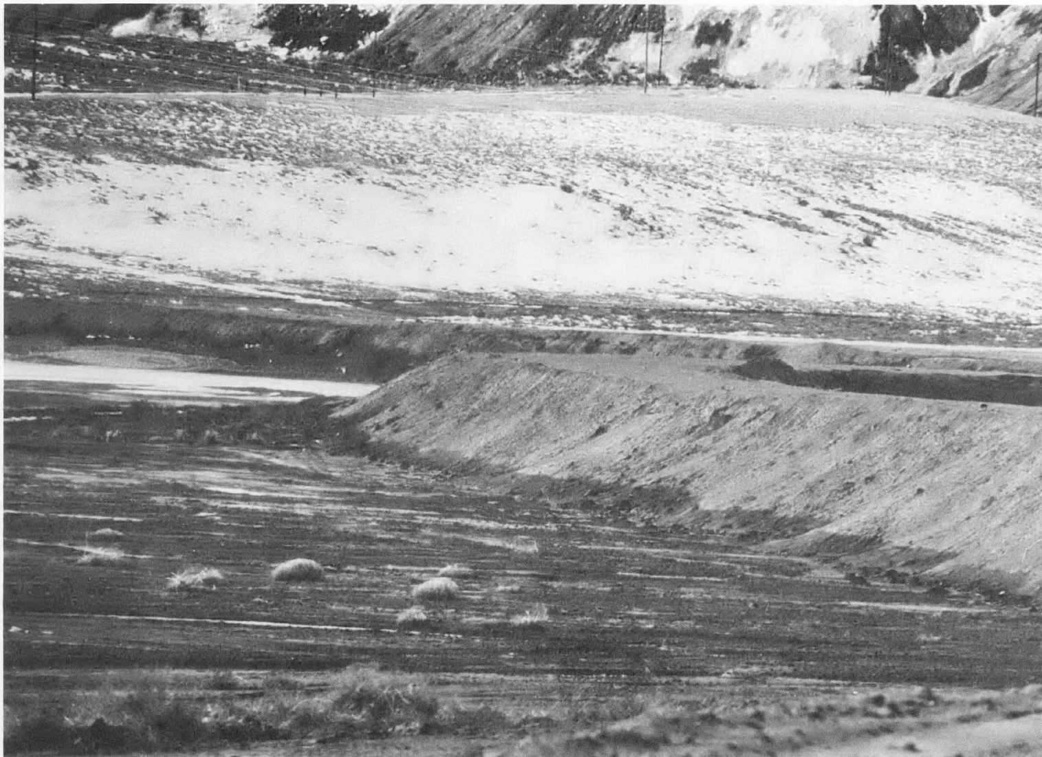
Figure 6-37. Dividing Berm, Naughton
