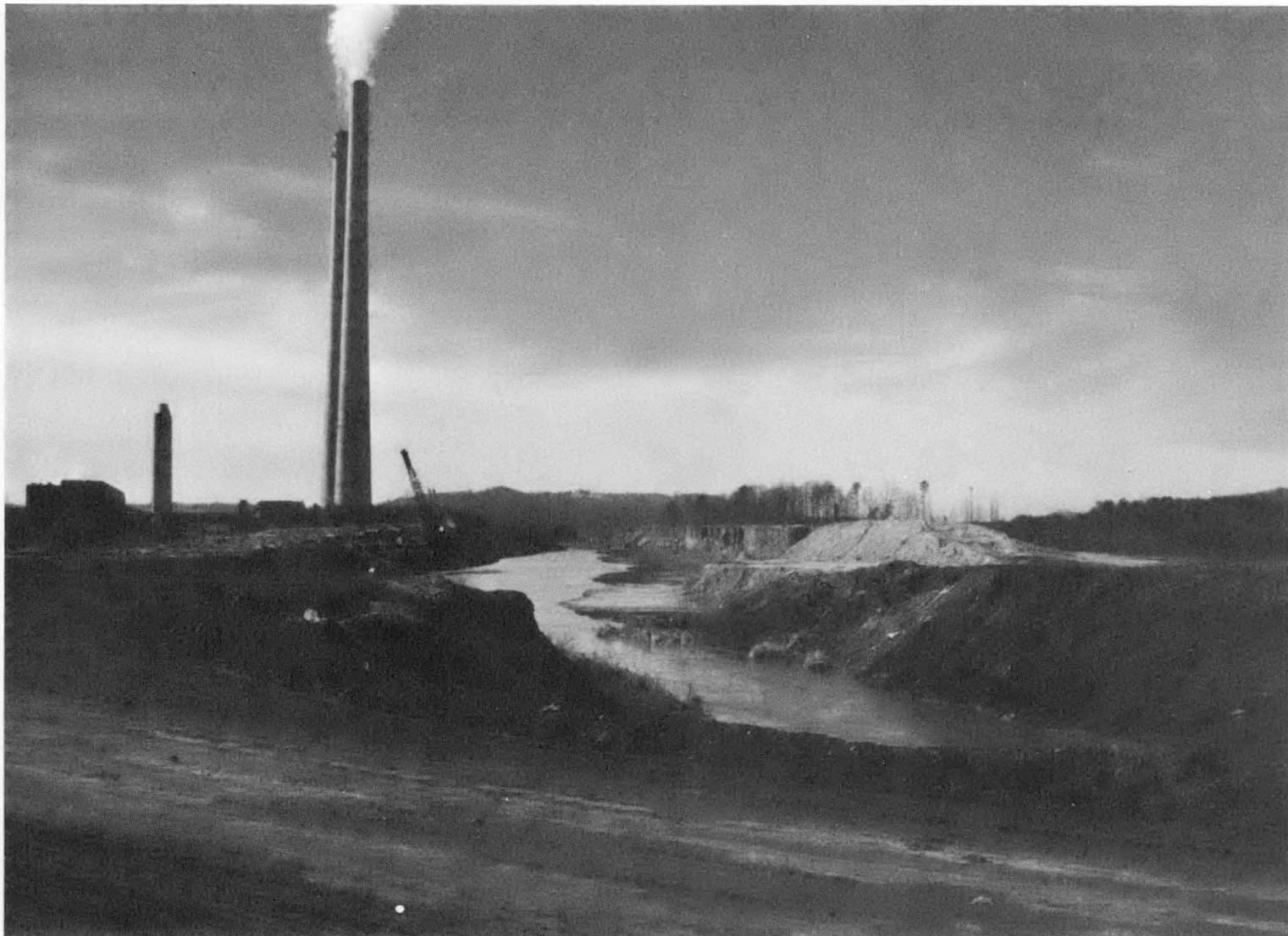
Figure 6-31. Bottom Ash Excavation, Kingston
