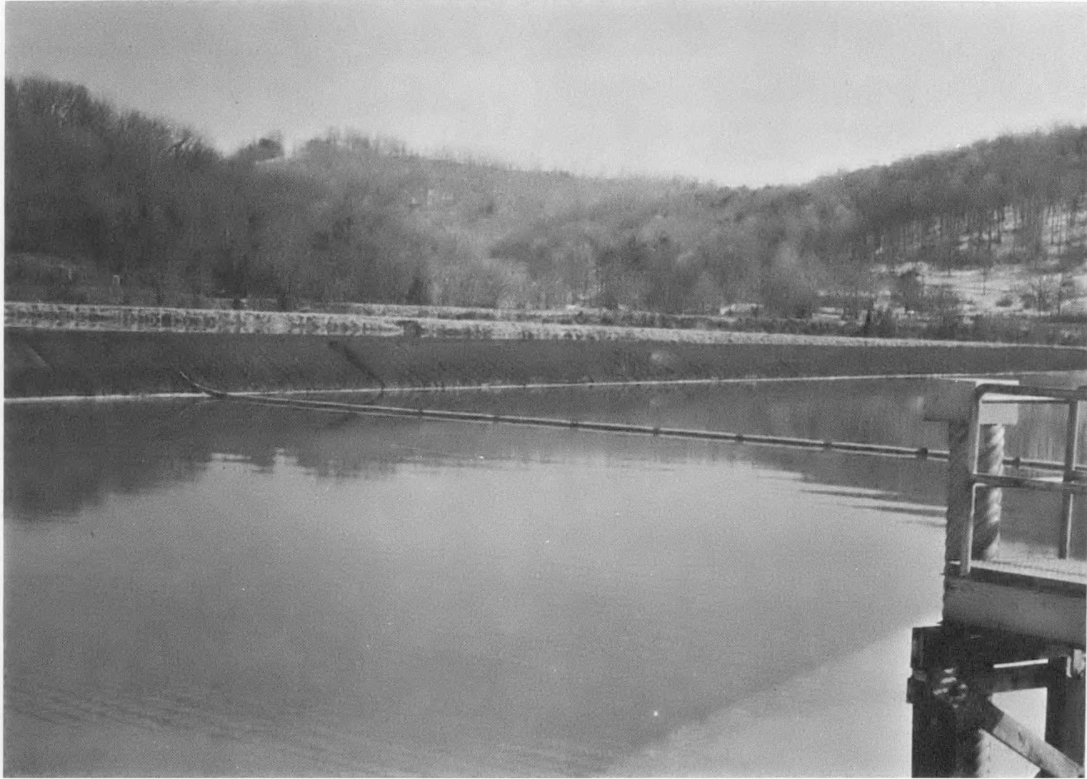
Figure 6-23. Ash Levee and Skimmer, Bull Run
