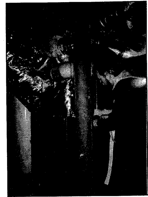
Property #4 - Heating System. Duct wrap insulation being installed to plenum.
