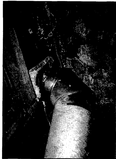
Property #6 - Disconnected ductwork. Duct connection before retrofitting.
