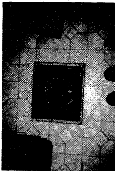
Property #3 - Poorly fitted register boot connection. Duct insulation filled the gaps around the boot.
