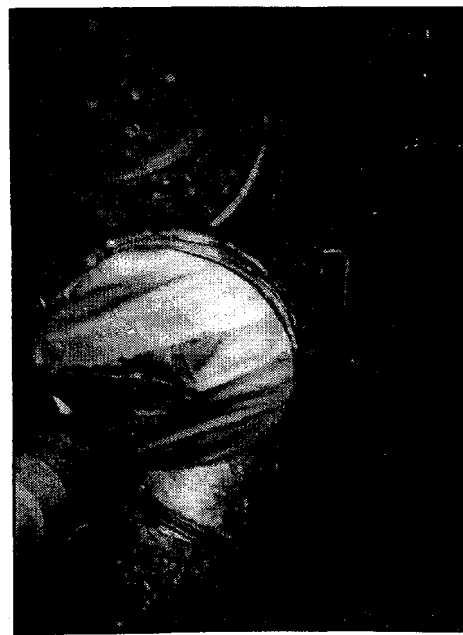
Property #7 - Ductwork sealed with duct tape.
