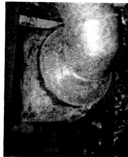
Property #3 - Loose register boot connection.
