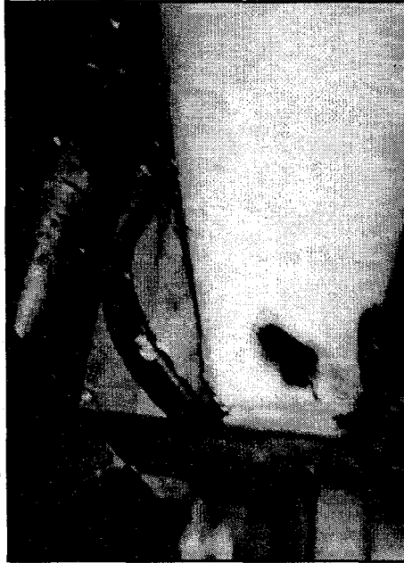
Property #5 - Disconnected ductwork; A-ttempts at insulating ductwork.
