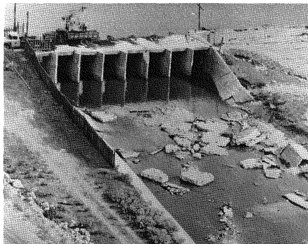
Figure 5—Spillway damage at Hebgen Dam. (Montana Power Company photo.)
