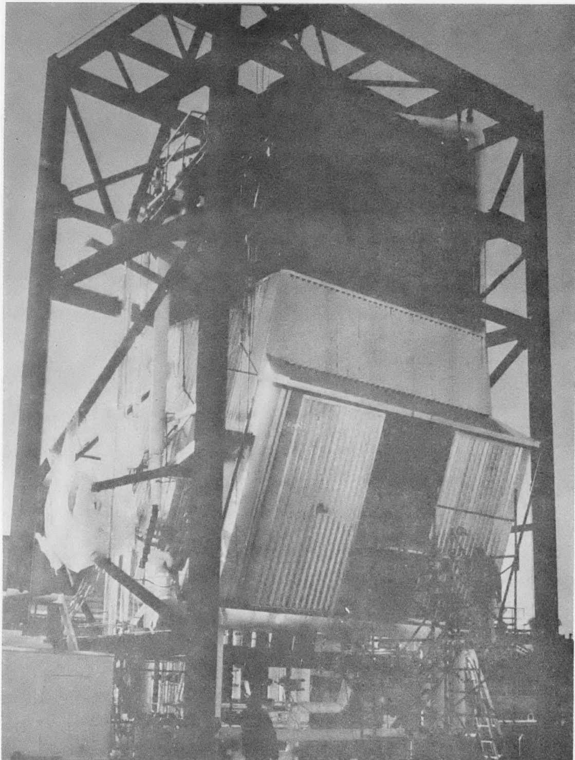
Figure III.F-4 SRE Receiver ( 5m_w_t ) Installed at STTF
