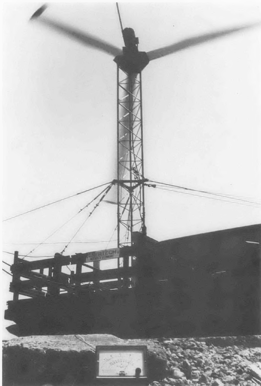
Figure 51 E-4000 Operating at an Indicated Wind Speed of 85 mph Mt. Washington, 5/21/80
