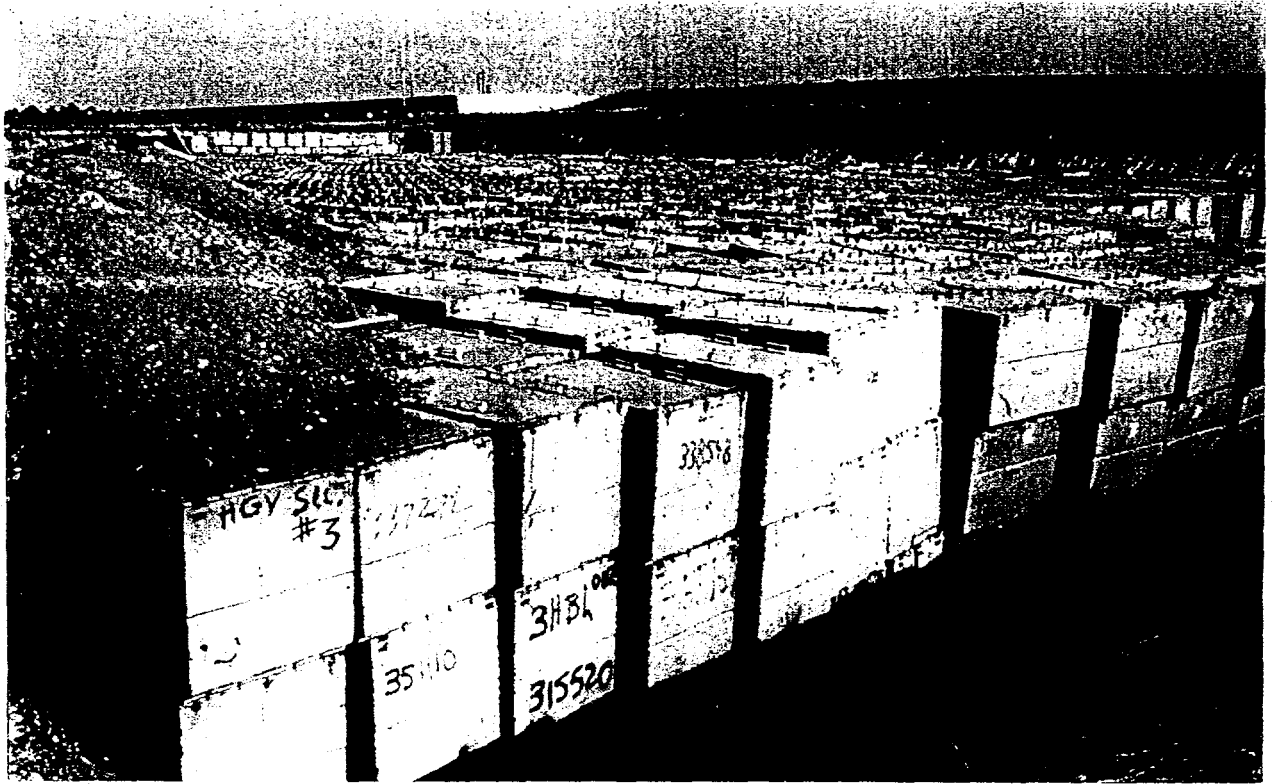
Figure 32. Engineered Trench for Low-Level Radioactive Waste. A trench like this in the Savannah River Site Solid Waste Disposal Facility may be used for disposal of the HWCTR reactor vessel and steam generators if they are removed during the decommissioning. Located in E-Area, this facility is approximately three miles from the HWCTR property.
