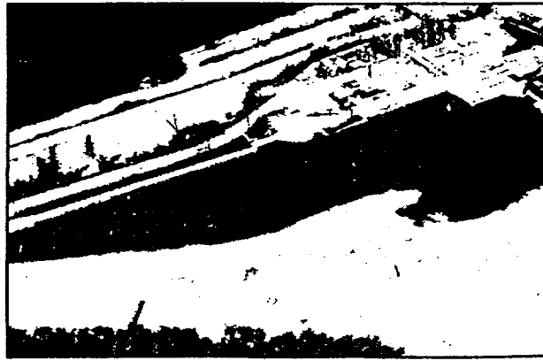
Figure 30. The Shippingport Decommissioning. These before and after views of the 7.5 acre property illustrate what is meant by the "greenfields" complete dismantlement type of nuclear reactor facility decommissioning.
