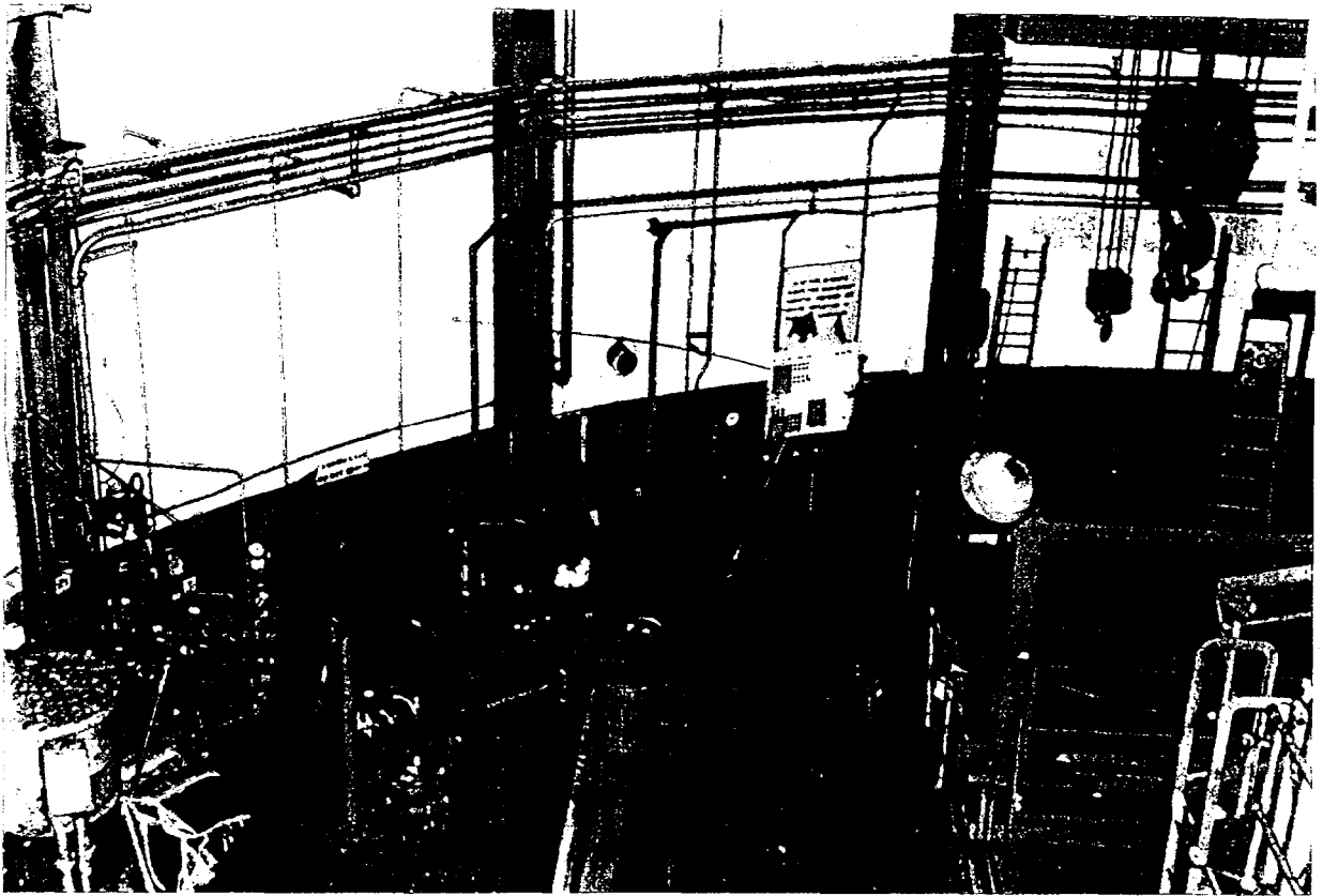
Figure 9. Part of the 0-Level Main Floor. Wooden planks covering the spent fuel basin can be seen on the right. Note the polar crane hook at upper right. During spent fuel handling in the basin, the hook was immersed in the basin water. The hook and crane cables remain radioactively contaminated.
