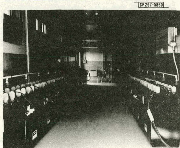
Fig. 4. 600-kWh storage battery at NBNM.
