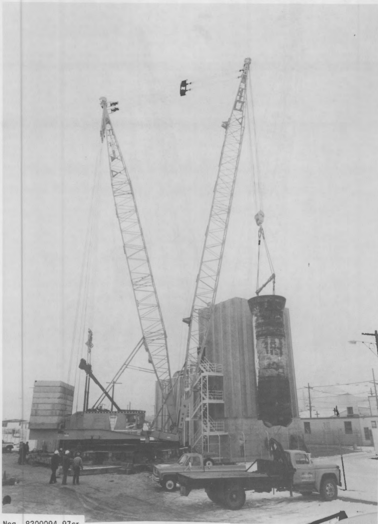
FIGURE 3. Lifting the Generator into the SGEF
