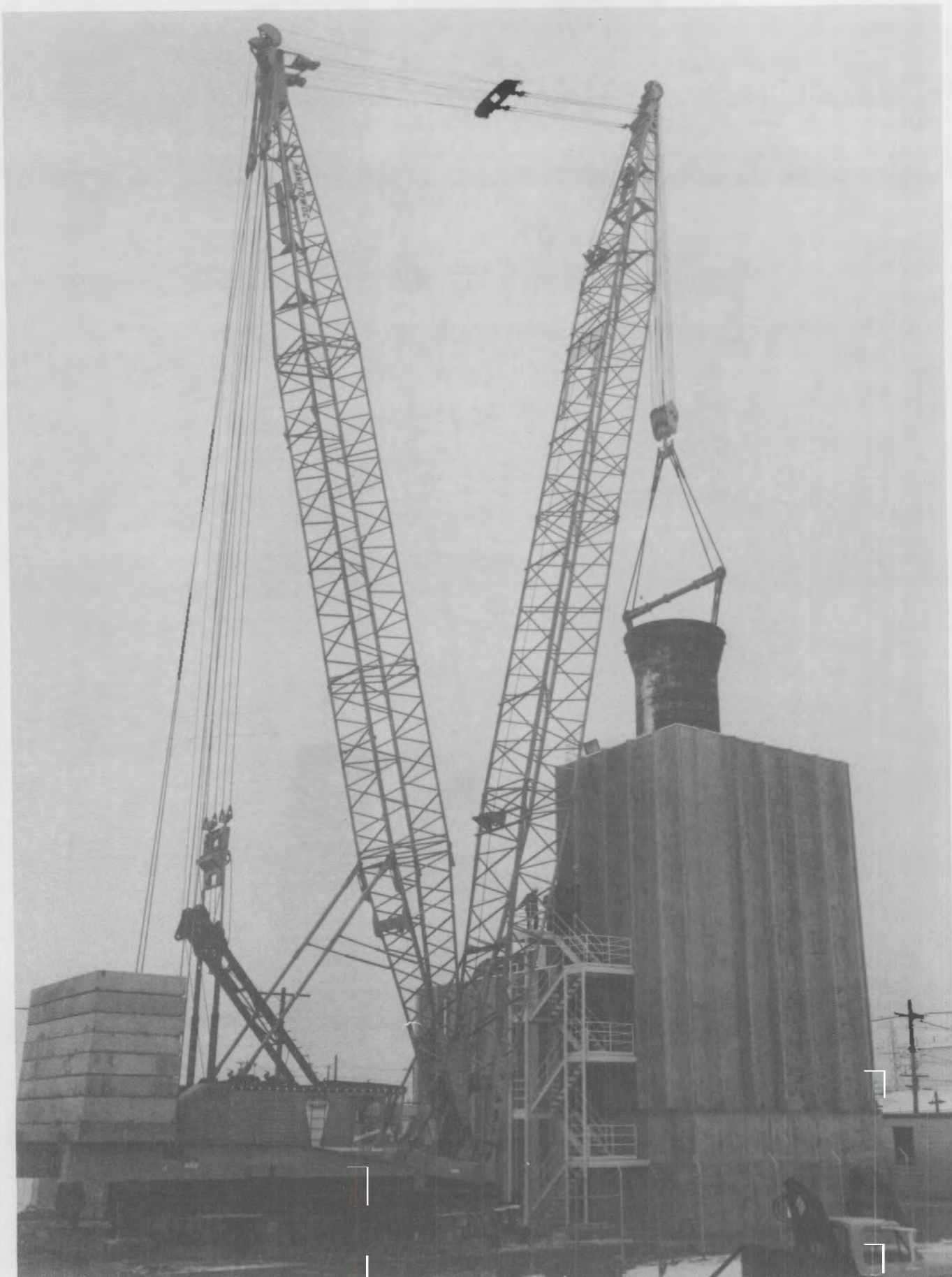
FIGURE 4. View of the Generator As It Entered the SGEF Through the Removable Roof Panel
