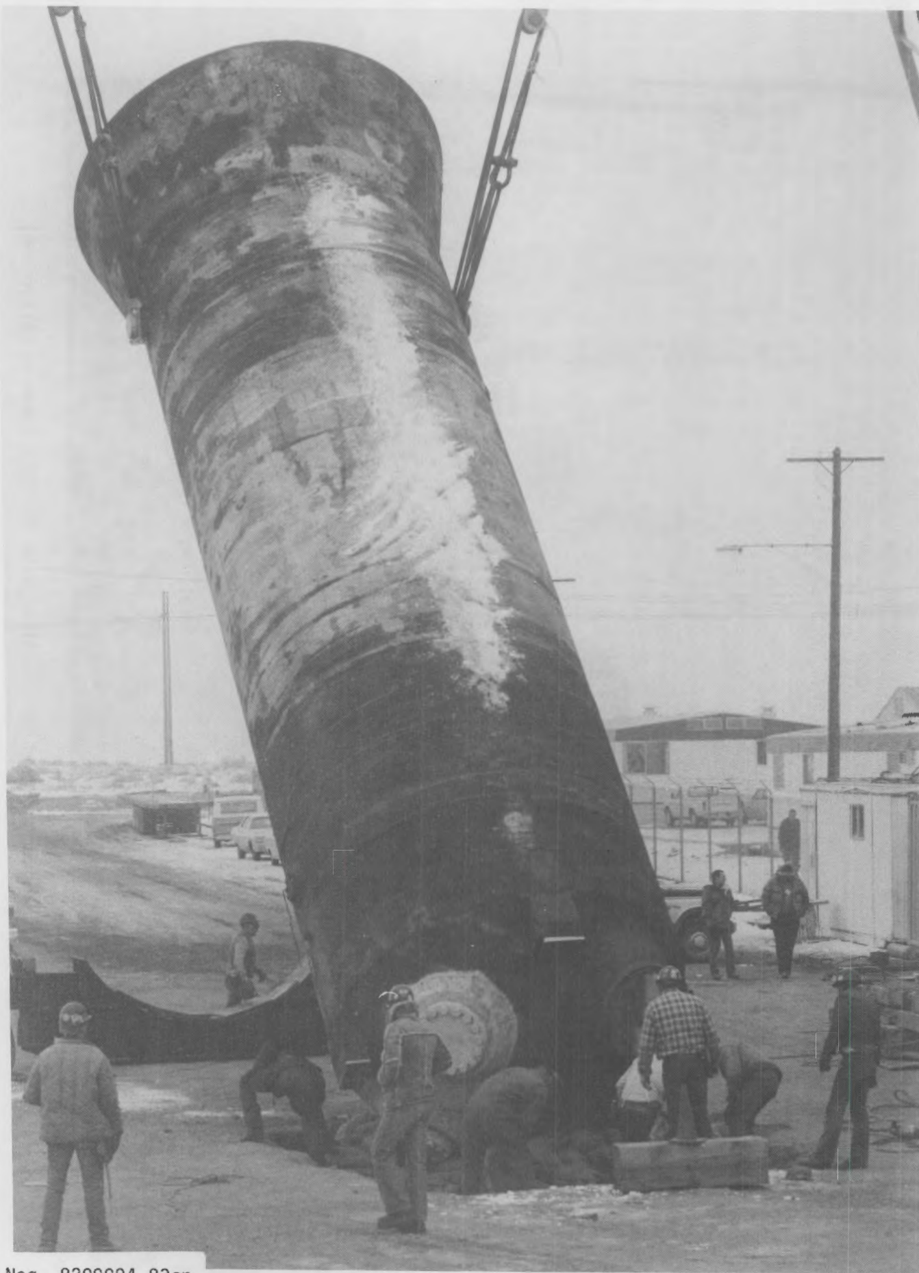
FIGURE 2. Tilting the Generator into a Vertical Position
