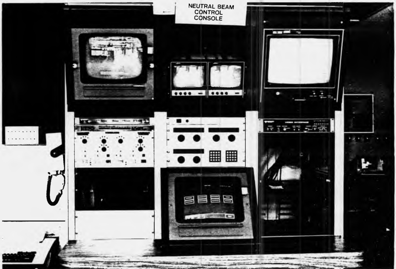
Fig. 2. Neutral beam console.
