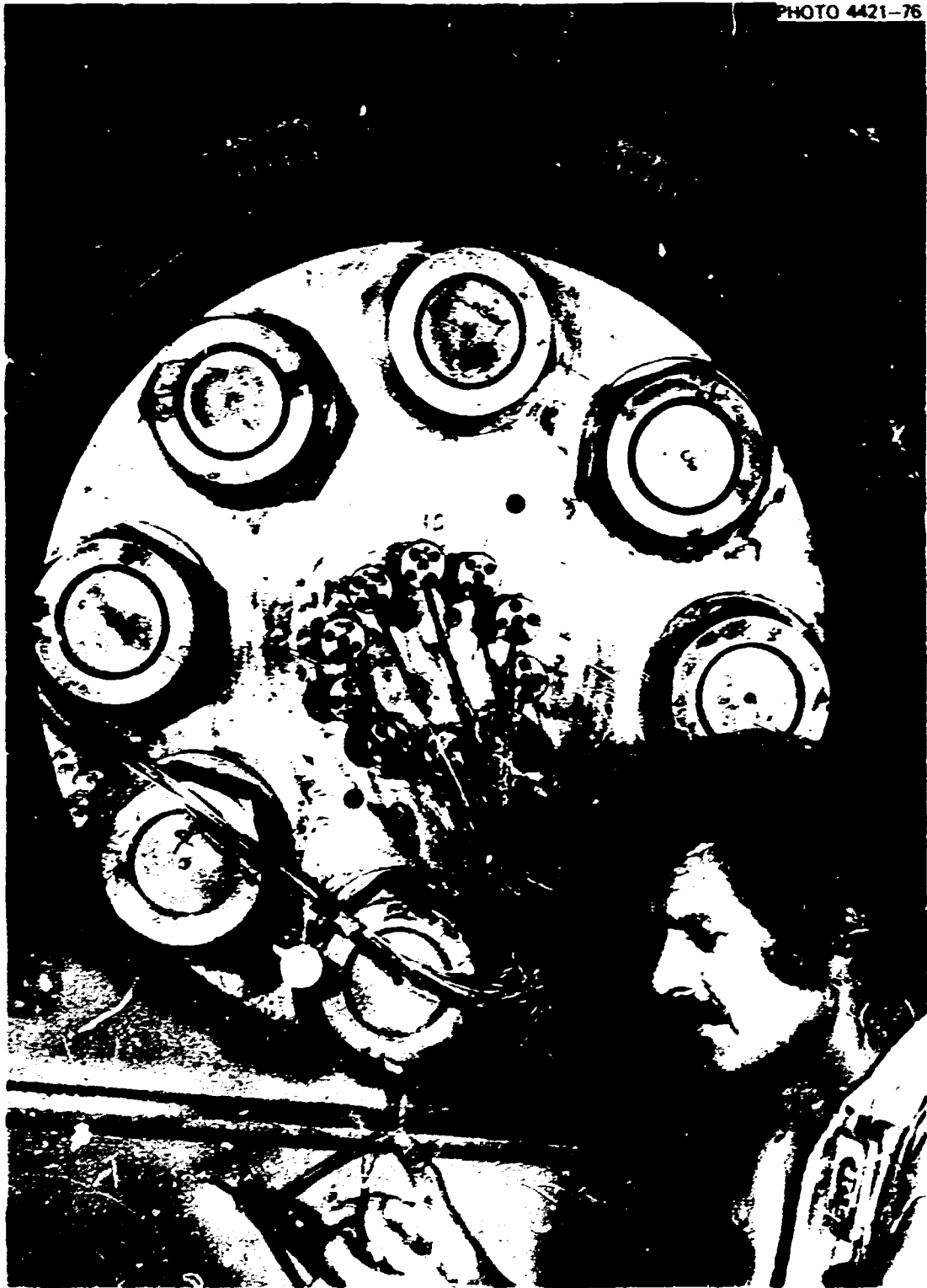
Fig. 4.11. Closure end view of V-7A vessel assembly showing Autoclave Engineers high-pressure penetration fittings for instrumentation cables.
