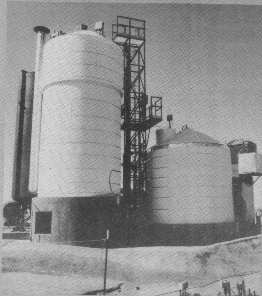
Figure 2-5 Thermal Storage Subsystem
