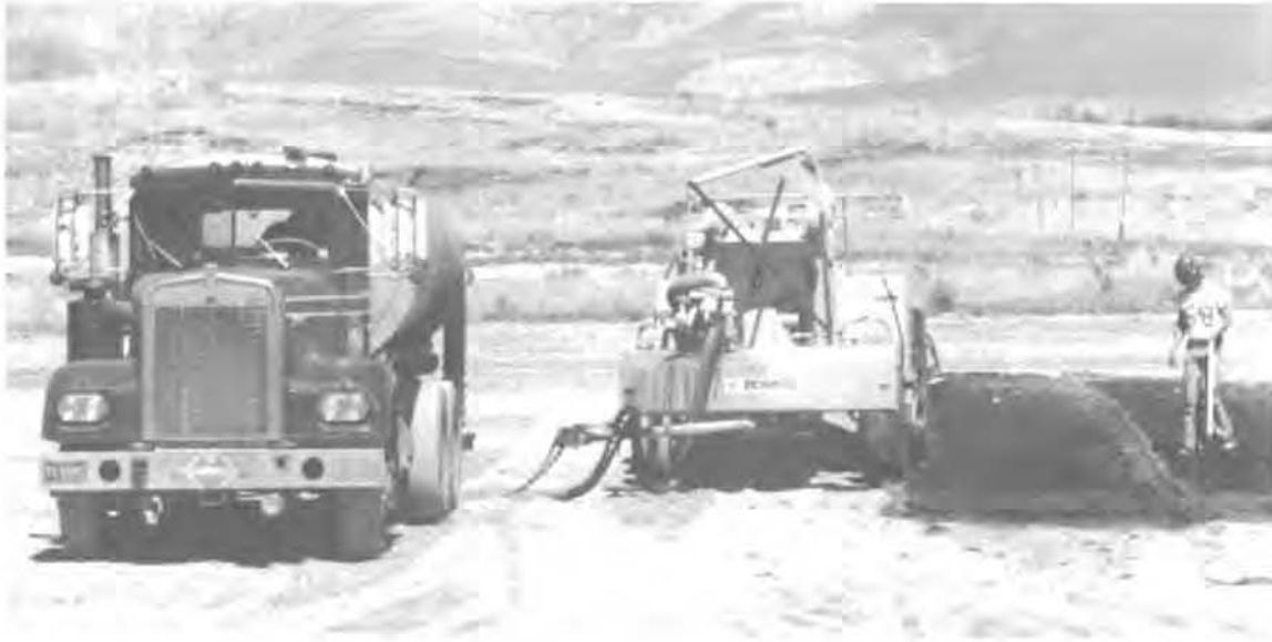
FIGURE 20. BOMAG MPH 100 and Distributor Truck Operating in Tandem
