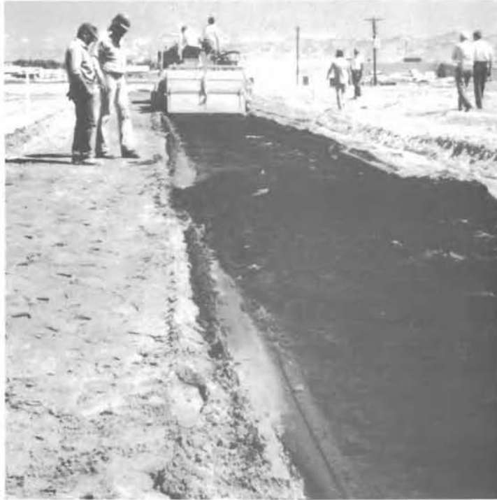
FIGURE 18. Preliminary Test of BOMAG MPH 100 Applying Asphalt Emulsion
