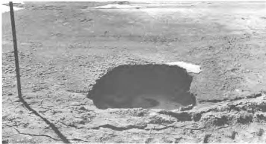
FIGURE 43. Sink Hole at North Edge of Area 7
