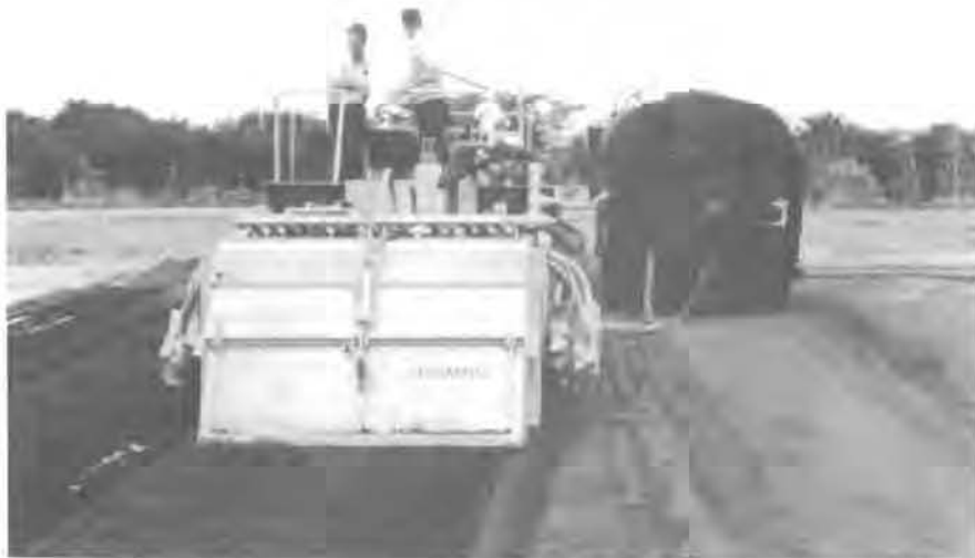
FIGURE 22. Second Application of \sim 9 wt% Asphalt Emulsion
