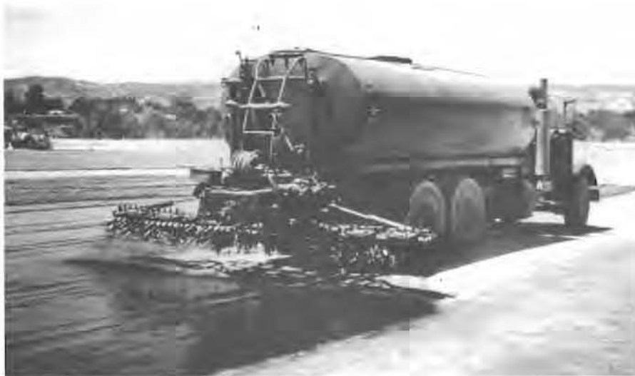
FIGURE 23. Applying the Spray-Coat Seal on the Admix Seal
