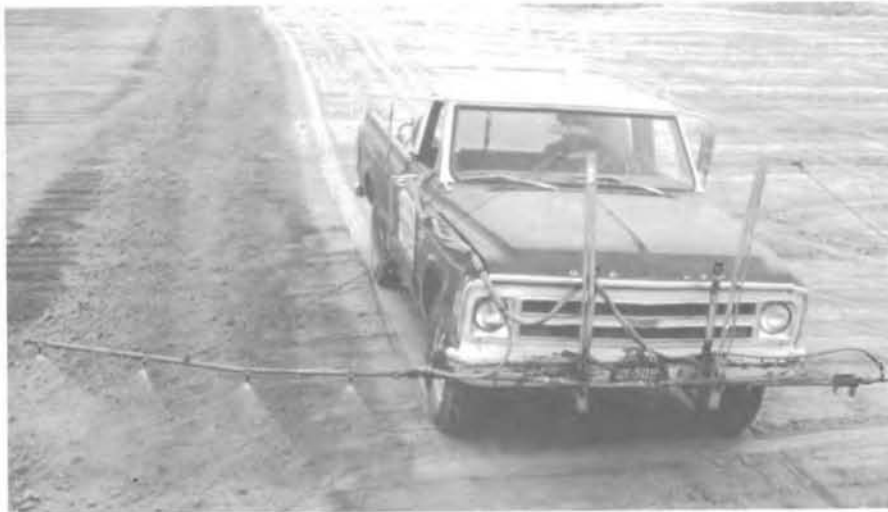
FIGURE 27. Herbicide (Treflan ® ) being applied to ~7.6 cm of Overburden on the Seal
