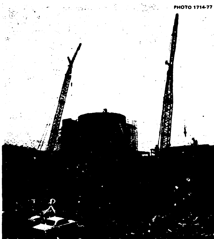
Fig. 1.2. Construction site on April 20, 1977. Concrete walls and roof of the first floor, which is predominantly below the elevation of the street, are complete. Steel structure for the remaining two floors is in place to the right of the tower. The corner of the gas-compressor building is shown on the right. This building will house two 450-hp compressors used in transferring the \text{SF}_6 and three \text{SF}_6 storage tanks.
