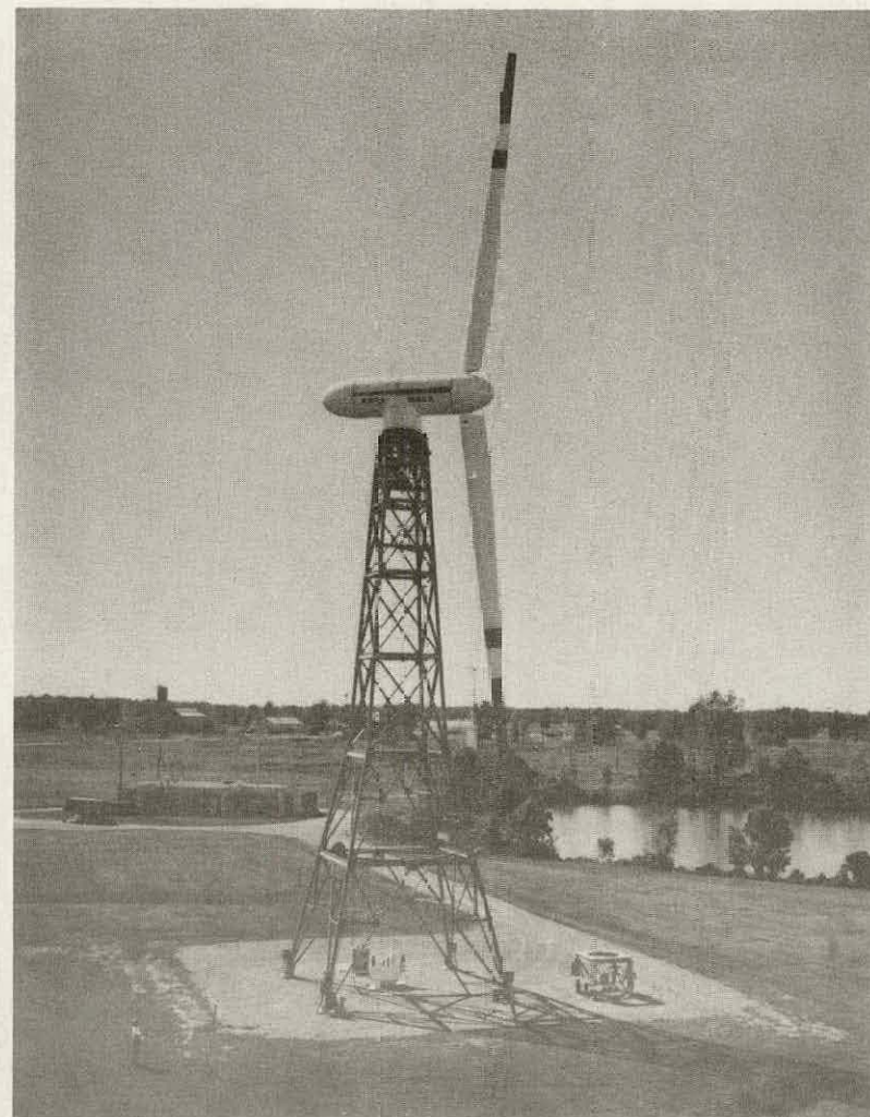
(b) Original configuration, with fully pitched aluminum blades and rigid hub.
